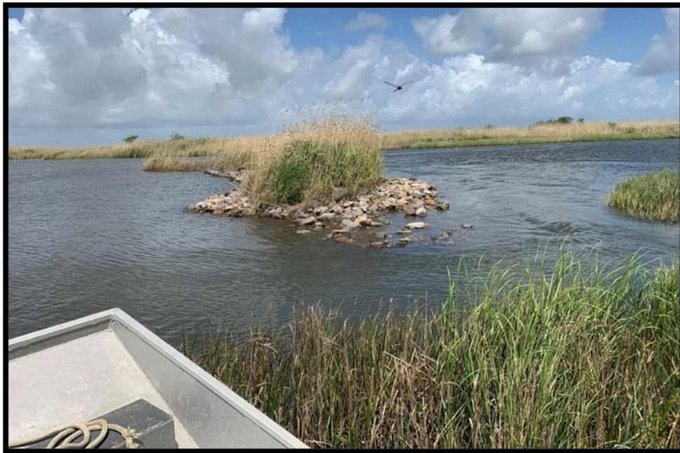
Figure 11. Mangrove Bayou Interior Canal Plug - Scouring of Eastern Tie-in, Post-Hurricane Laura
