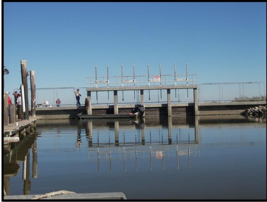
Figure 8. No Name Bayou Water Control Structure, Pre-Hurricane Laura
