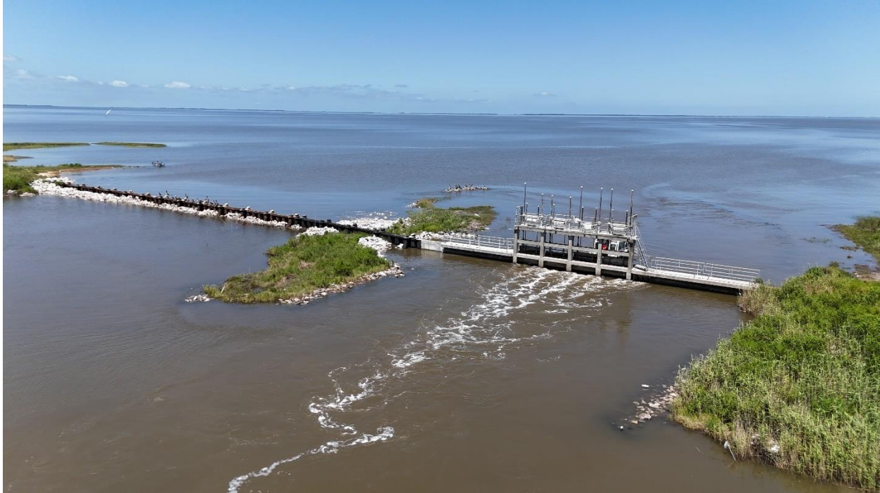
Figure 23. Lambert Bayou Breach and Water Control Structure, Post-Construction
