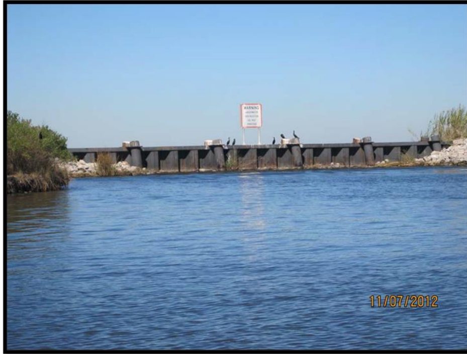
Figure 6. Grand Bayou Levee Breach Structure, Pre-Hurricane Laura
