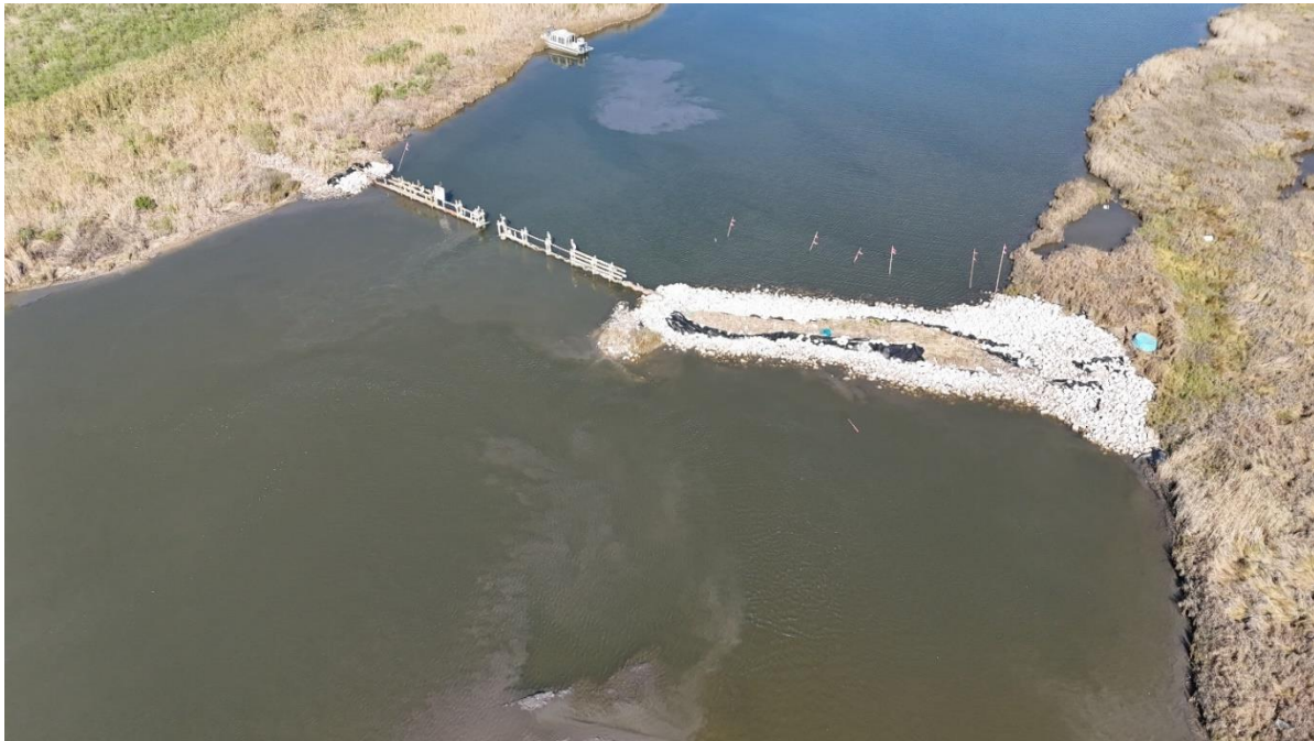
Figure 19. Mangrove Bayou Interior Canal Plug, Post-Construction
