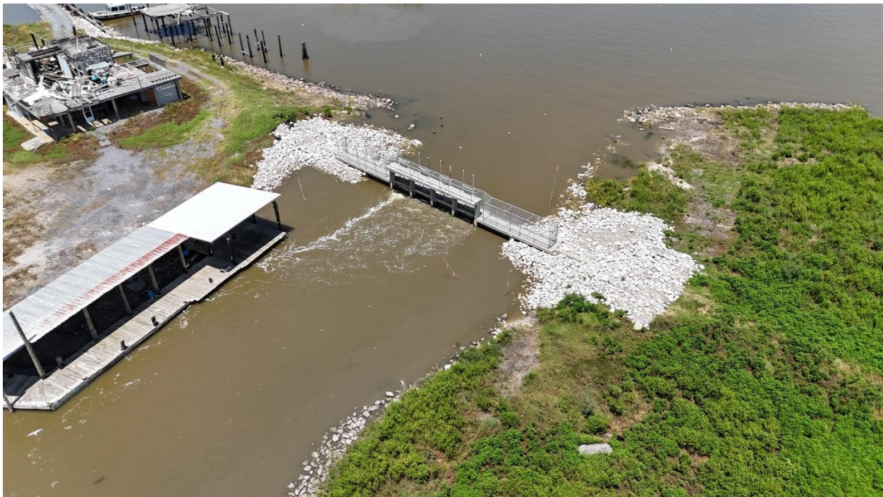
Figure 24. No Name Bayou Water Control Structure, Post-Construction
