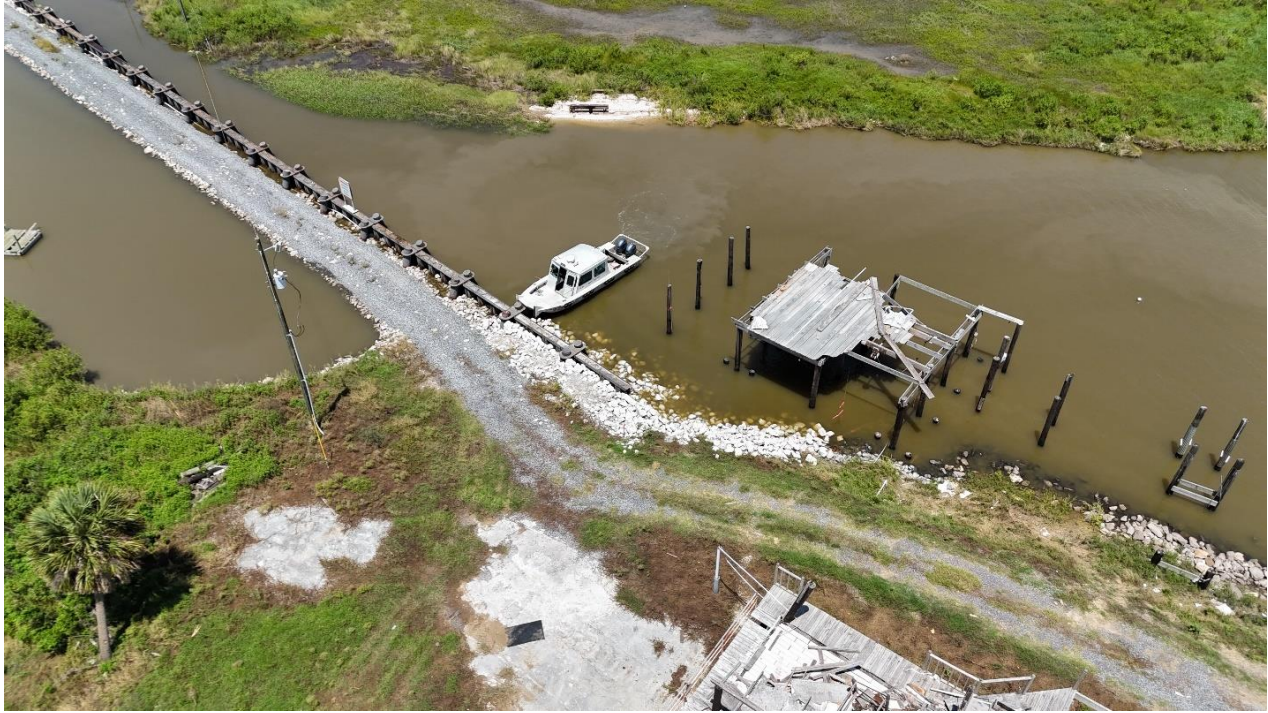
Figure 25. No Name Bayou Levee Breach Structure, Post-Construction
