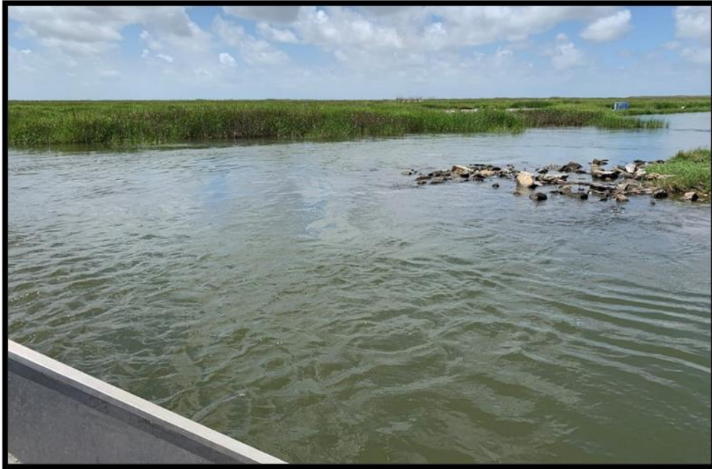
Figure 12. Grand Bayou Interior Canal Plug - Scouring of Eastern Tie-In, Post-Hurricane Laura
