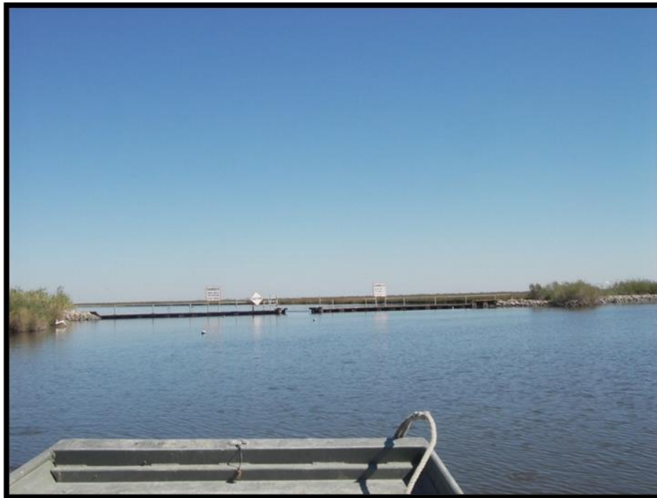
Figure 3. Mangrove Bayou Interior Canal Plug, Pre-Hurricane Laura
