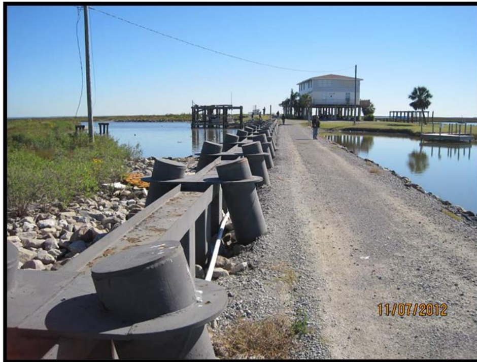
Figure 9. No Name Bayou Levee Breach Structure, Pre-Hurricane Laura
