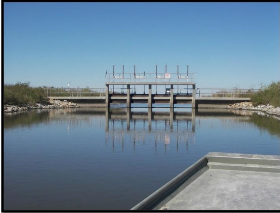
Figure 2. Mangrove Bayou Water Control Structure, Pre-Hurricane Laura
