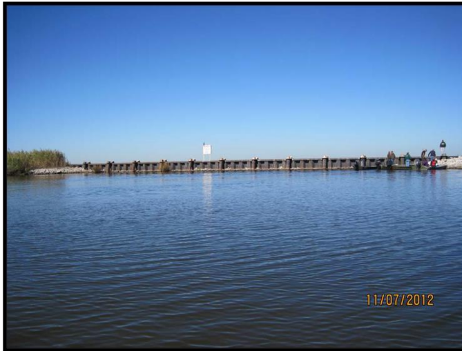
Figure 7. Lambert Bayou Levee Breach Structure, Pre-Hurricane Laura
