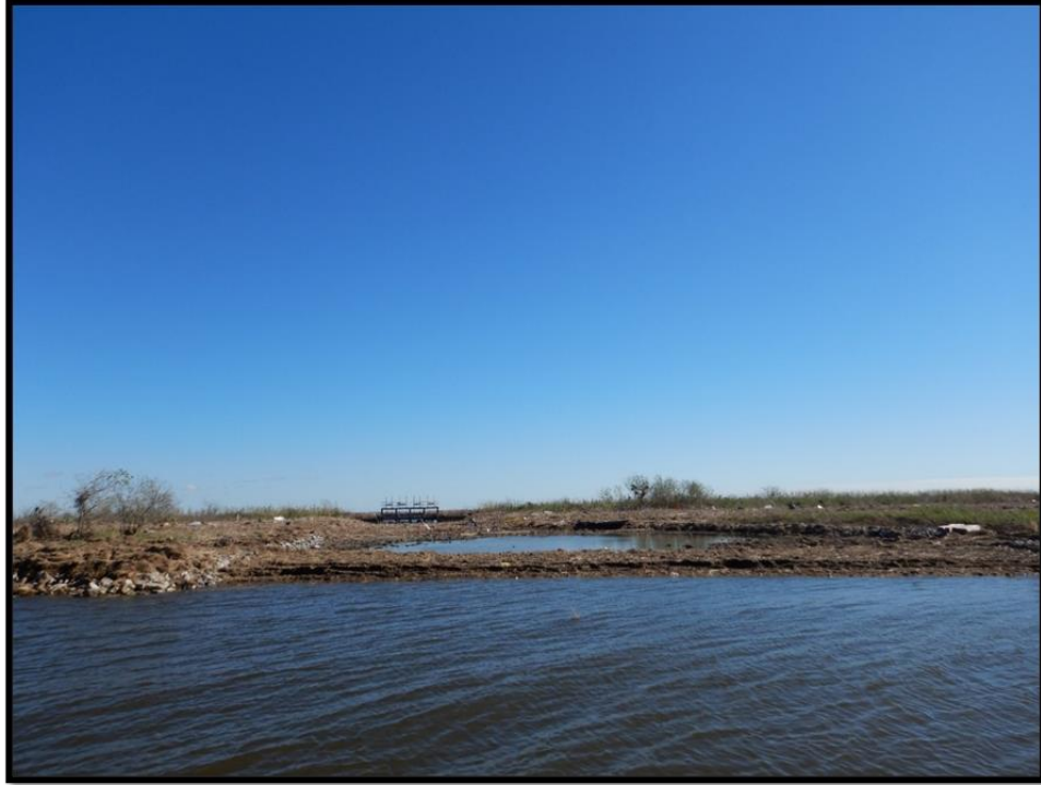
Figure 10. Mangrove Bayou Outlet Channel- Siltation & Debris, Post-Hurricane Laura
