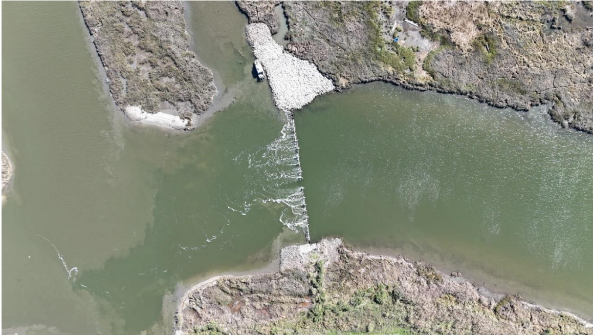
Figure 20. Grand Bayou Interior Canal Plug, Post-Construction
