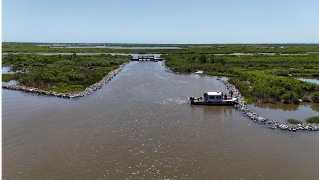
Figure 18. Mangrove Bayou Outlet Channel, Post-Construction
