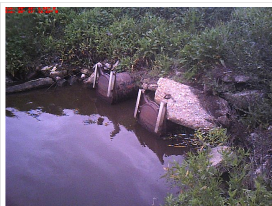
Flap Gates on Flood Side of Pump Station
