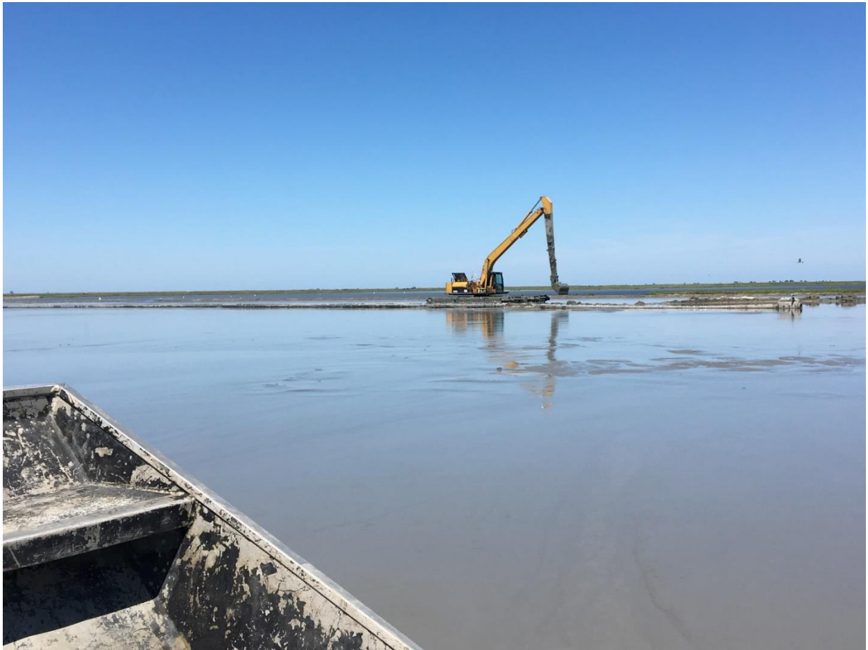
Figure 14: CS-54 Southern MCA Dredge Discharge Pipe and Track Hoe (4-10-2019).
