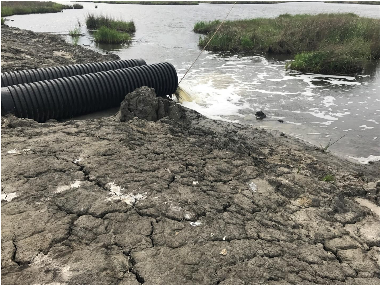
Figure 16. CS-54 Dewatering Culverts Flowing Southward Out of MCA.
