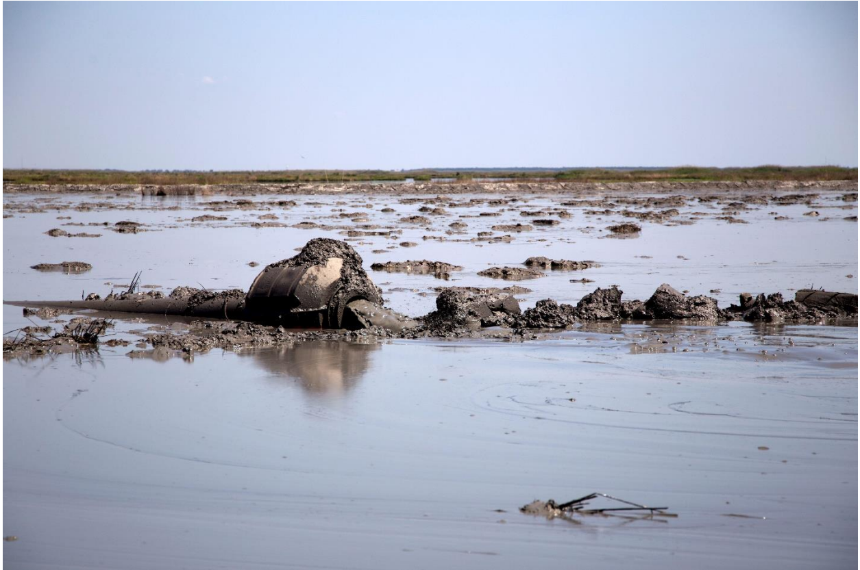
Figure 6: CS-54 Dredge Discharge into North MCA 2 months prior to MCA completion (5-9-2018).
