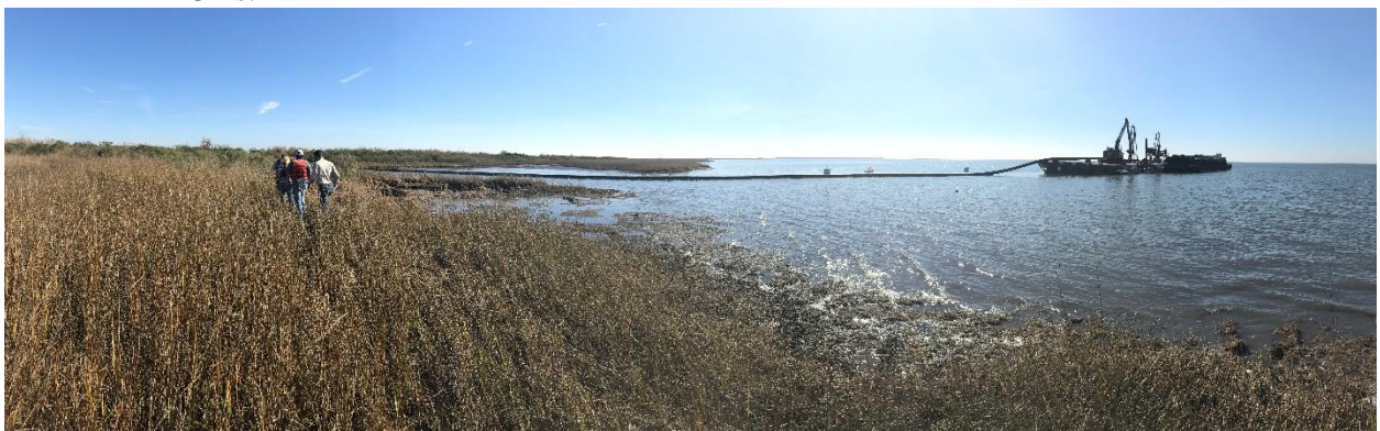
Figure 5: CS-54 Dredge Barge and Pipeline to the eastern Calcasieu Lake shoreline and MCAs.
