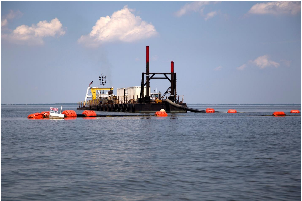
Figure 5: CS-54 Dredge Barge and Pipeline to the eastern Calcasieu Lake shoreline and MCAs.
