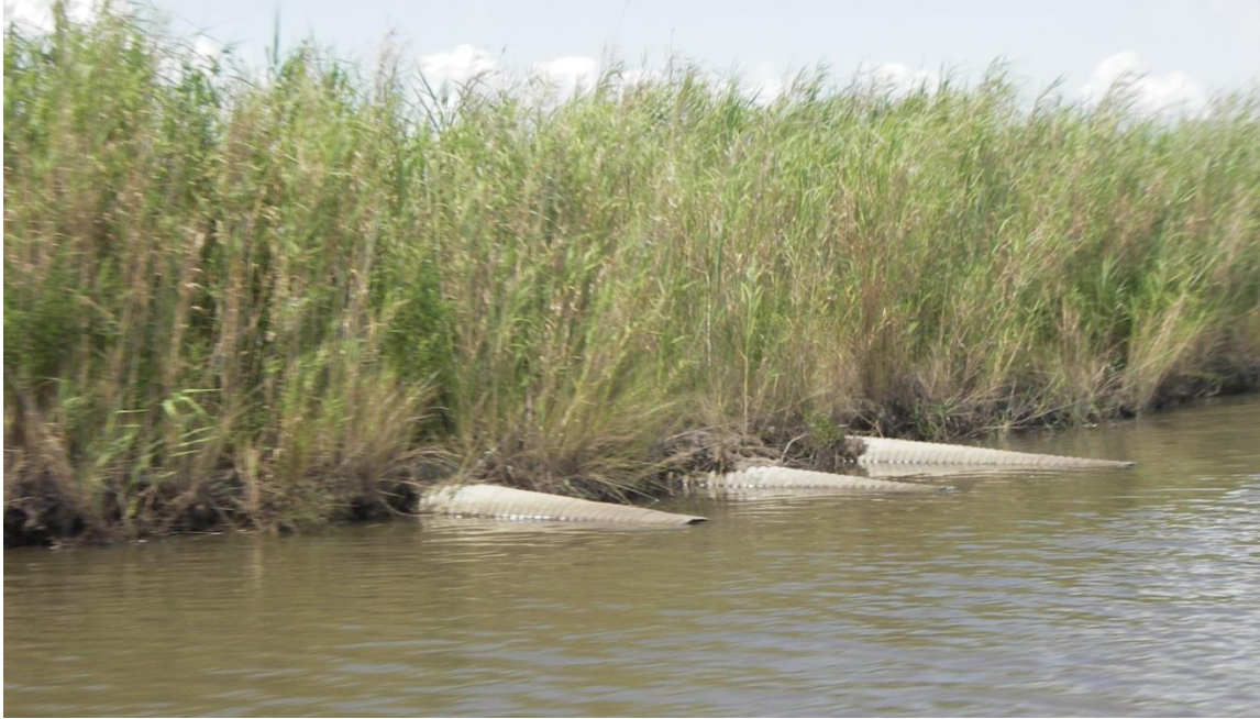
Photo No. 14 – Bridge Bayou Culverts in Grey’s Ditch (2016)
