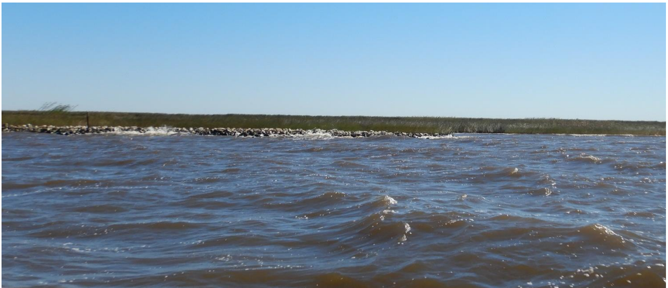
Photo No. 6 – South End of Sabine Lake Foreshore Rock Dike
