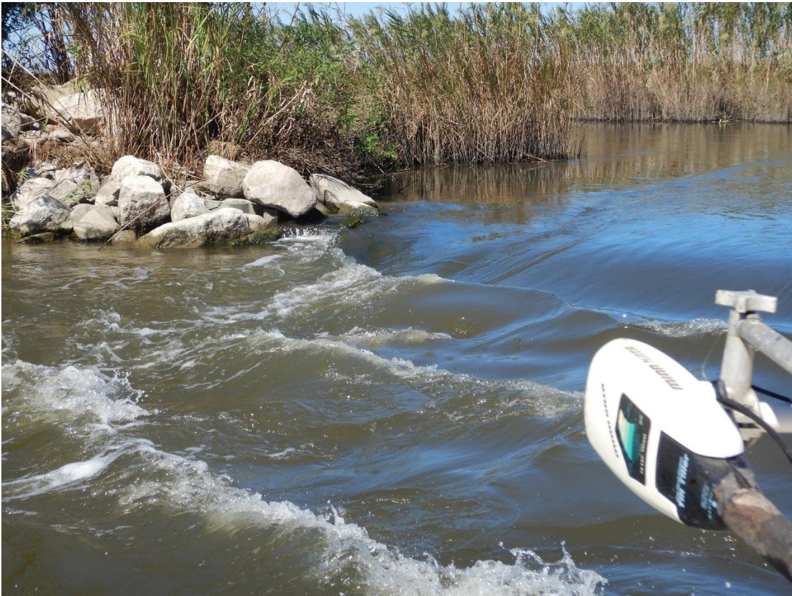
Photo No. 13 – Pines Ridge Weir, from Project Exterior
