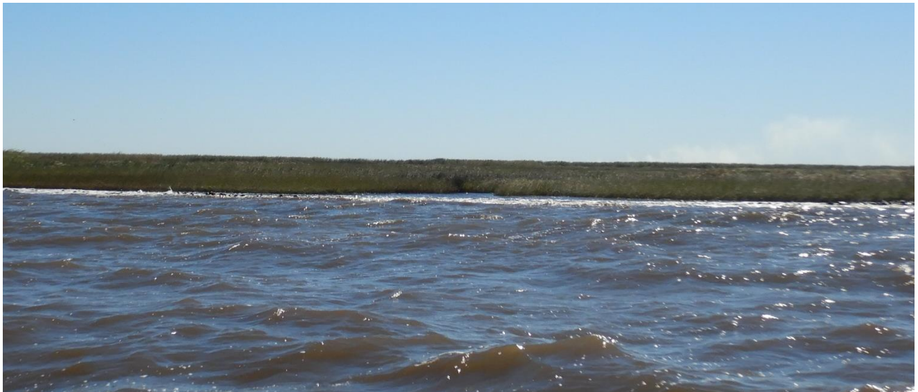
Photo No. 9 – Sabine Lake Foreshore Rock Dike, Low area of Rock
