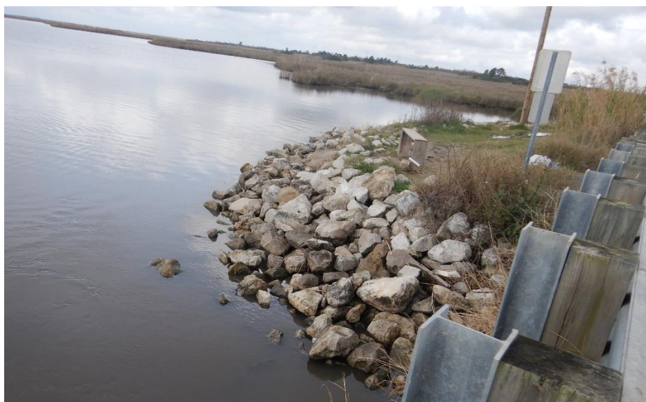
Photo No. 2, West Side (Looking North) – Rip Rap on North Bank of the Channel- January 2020
