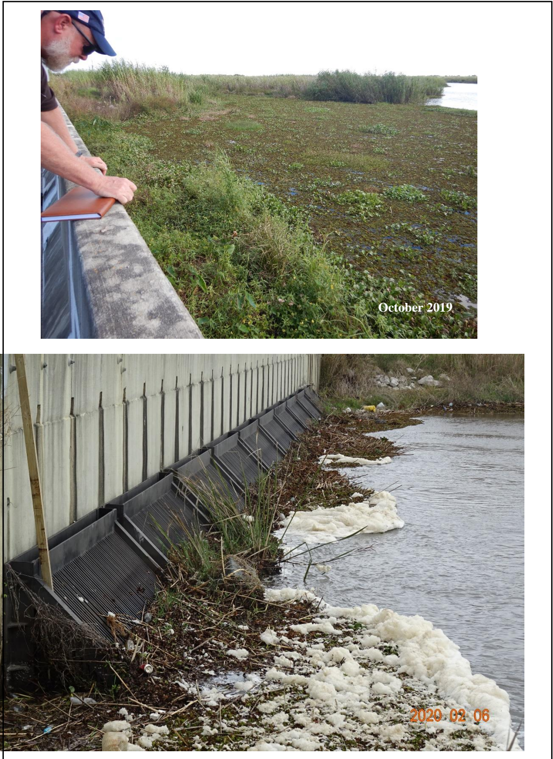
Photo No. 7, East Side of Box Culvert Structure (looking North), Trash Screens, Vegetation & Debris (October 2019 & February 2020)
