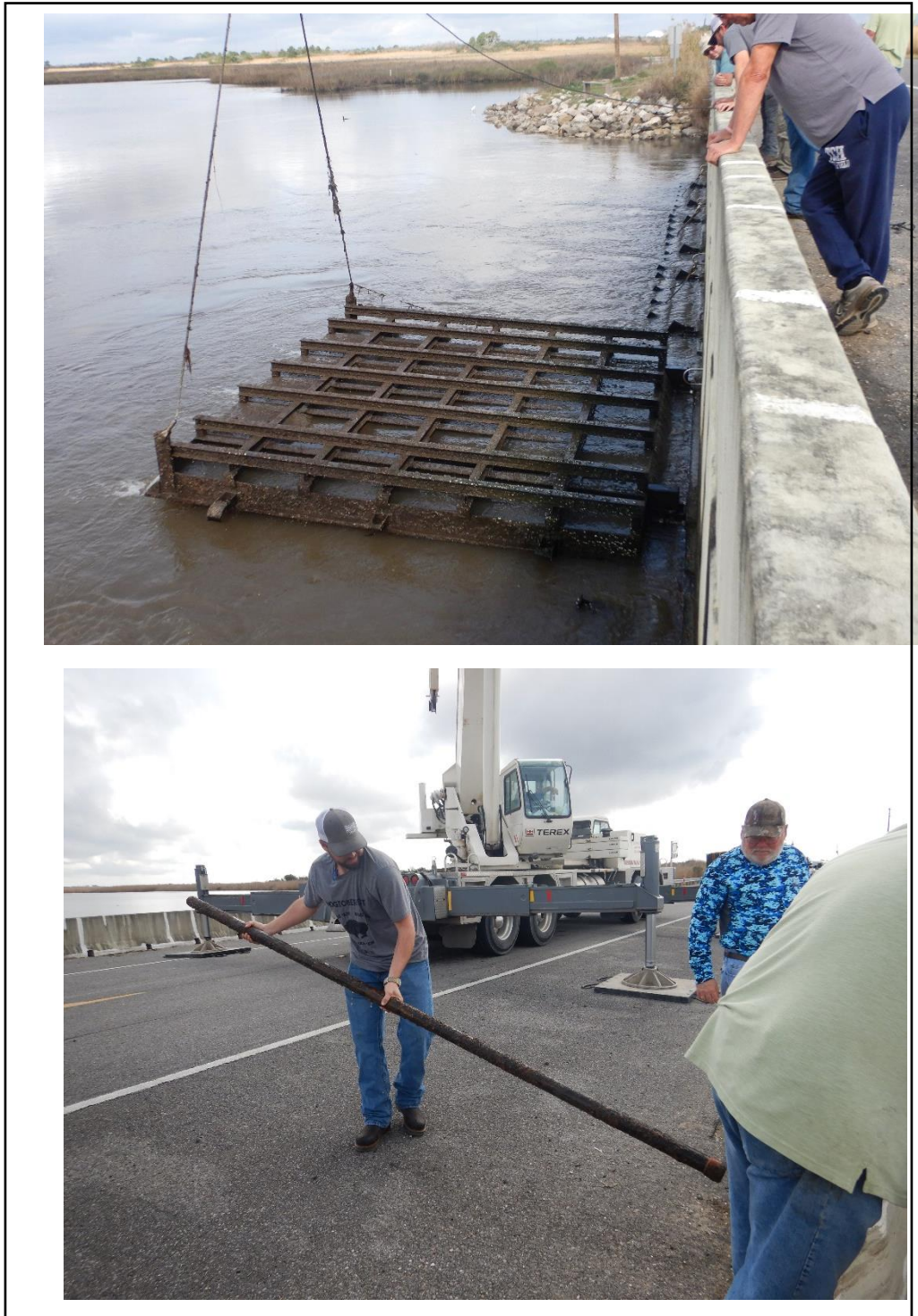
Photo No. 6, West Side of Box Culvert Structure, Flap Gate No. 4 – Broken Locking Rings & Steel Drill Pipe - January 2020
