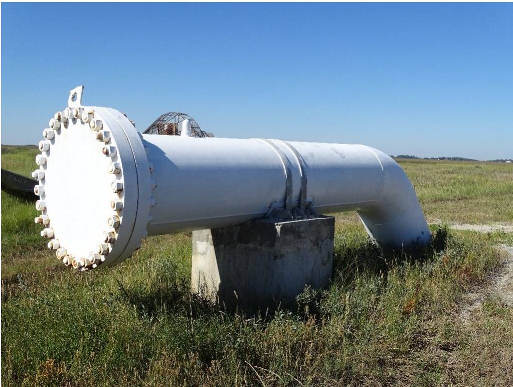
Photo No. 2, East end blind flange and riser (looking Southwest)
