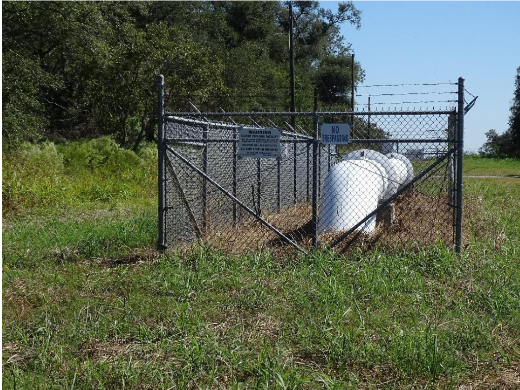
Photo No. 13, West Booster Station – looking East
