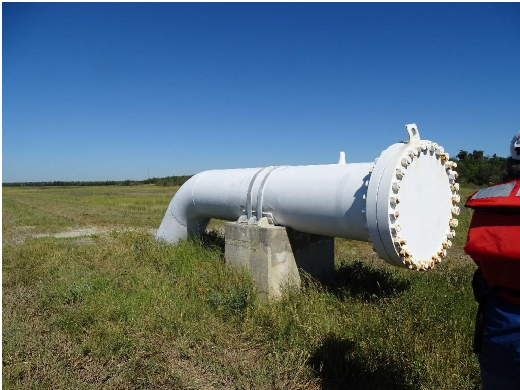
Photo No. 4, East end blind flange and riser (looking Northwest)
