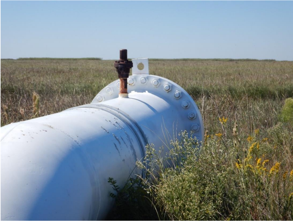
Photo No. 19, West Blind Flange and Riser looking South West
