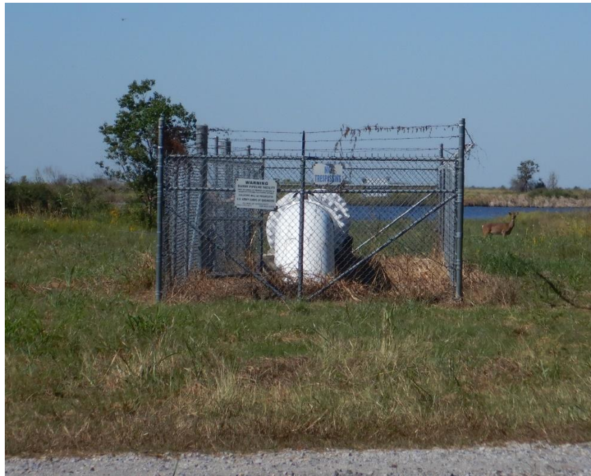
Photo No. 12, West Booster Station – looking west
