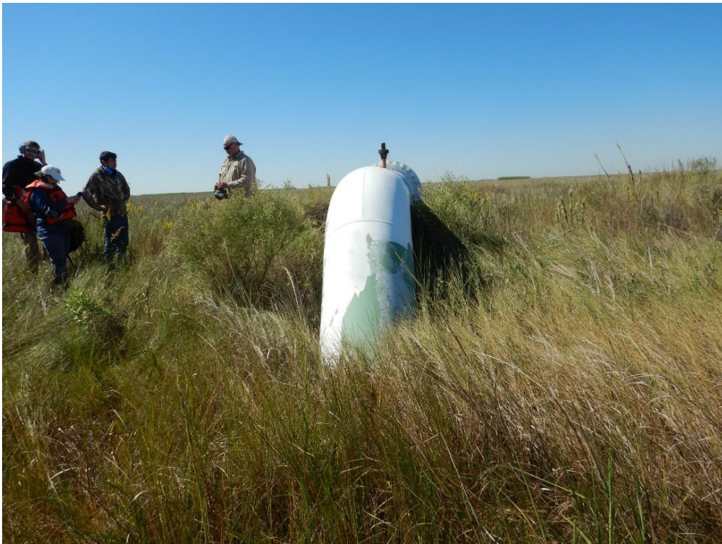
Photo No. 18, West Blind Flange and Riser looking West
