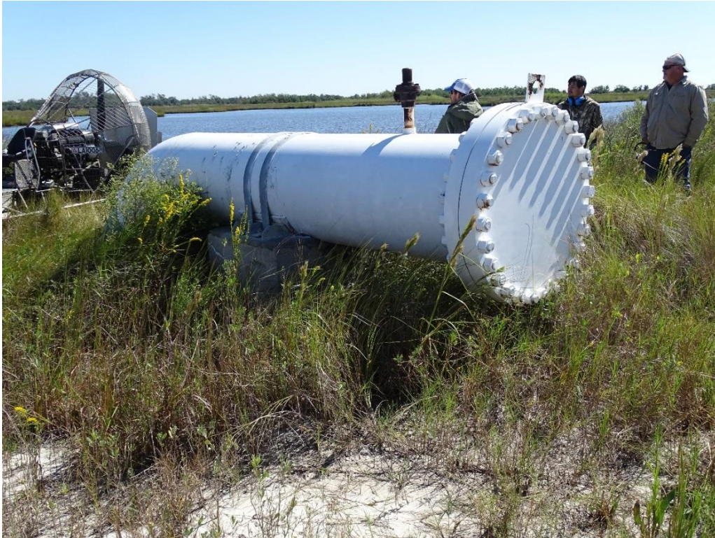
Photo No. 17, West Blind Flange and Riser looking South East
