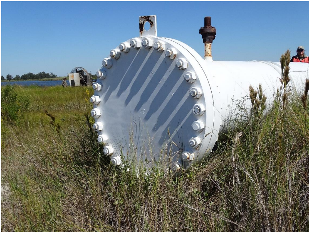
Photo No. 16, West Blind Flange and Riser looking North East
