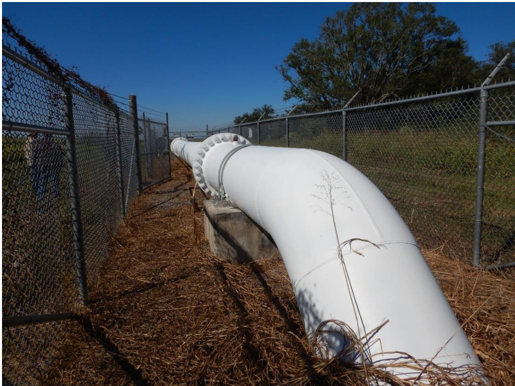
Photo No. 14, West Booster Station – looking West
