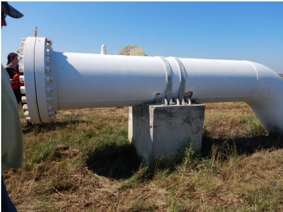
Photo No. 4, East end blind flange and riser (Looking Southward)
