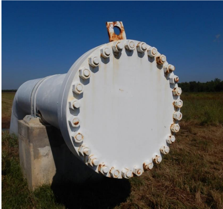
Photo No. 1, East end blind flange and riser (looking Westward)
