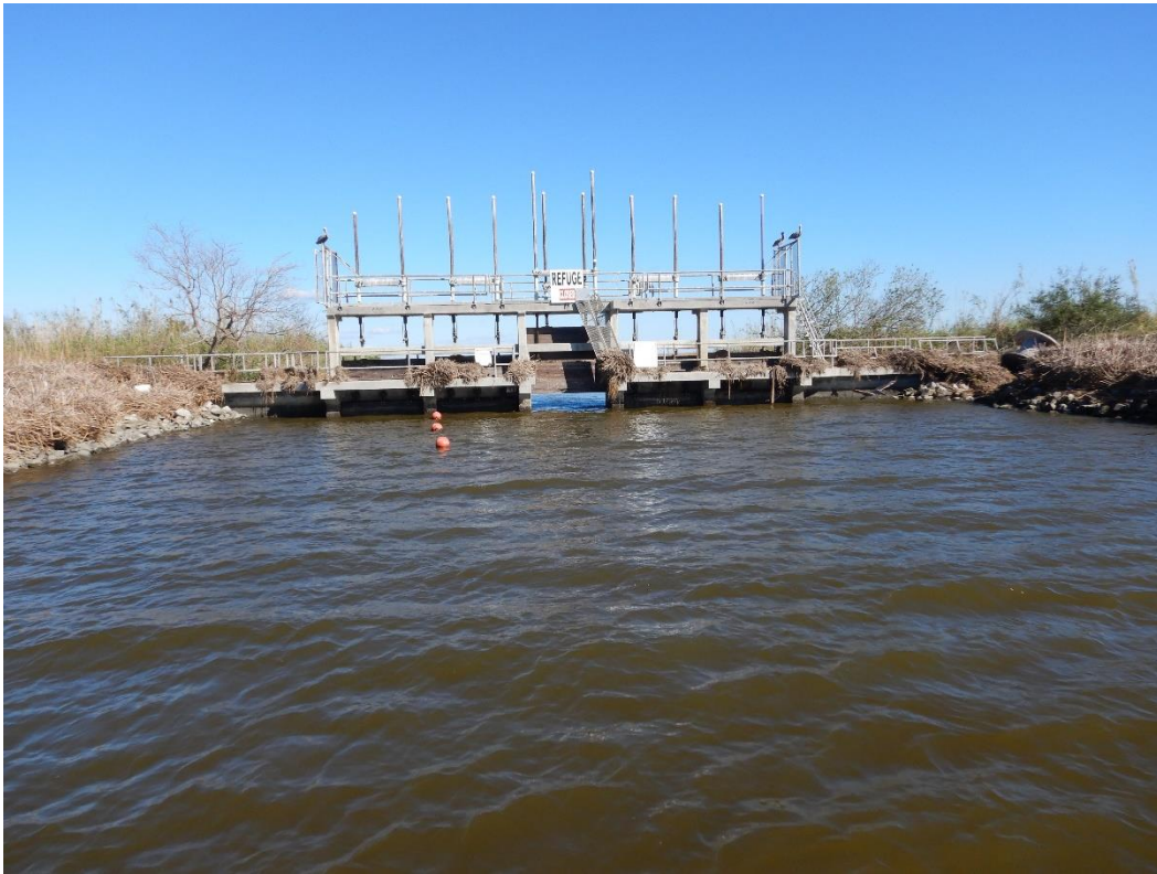
Photo No. 5, Grand Bayou Water Control Structure – Minor erosion and scour around end of structure.
