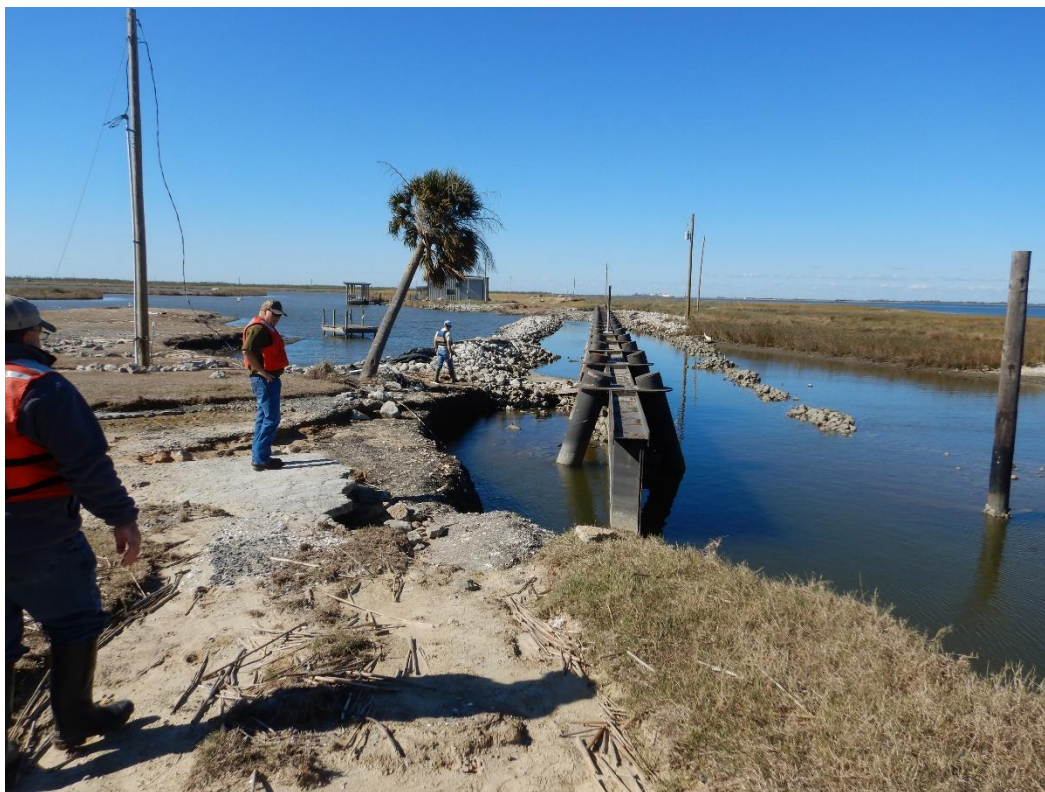
Photo No. 11. No Name Bayou Breach – Scour along and on ends of post Rita sheet pile repair.
