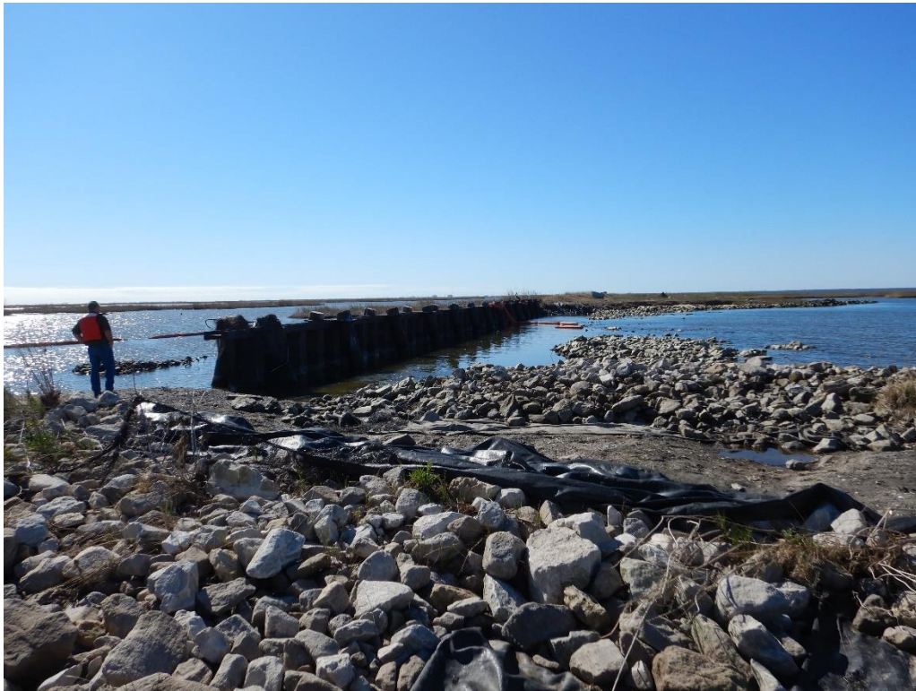
Photo No. 9. Lambert Bayou Breach – Scour on northern end and along sheet pile structure.
