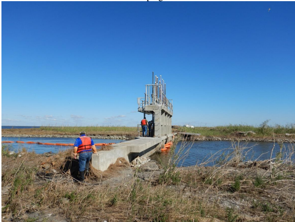
Photo No. 8. Lambert Bayou Water Control Structure – some scour and erosion on the land bridge connecting the water control structure to the sheet pile breach.
