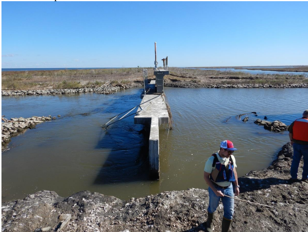
Photo No. 10. No Name Bayou Water Control Structure – Significant scour on each end of the structure.
