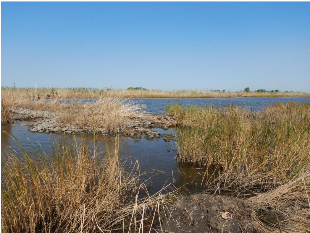
Photo No. 4. Mangrove Bayou Canal Plug – Erosion and scour on east side of structure.
