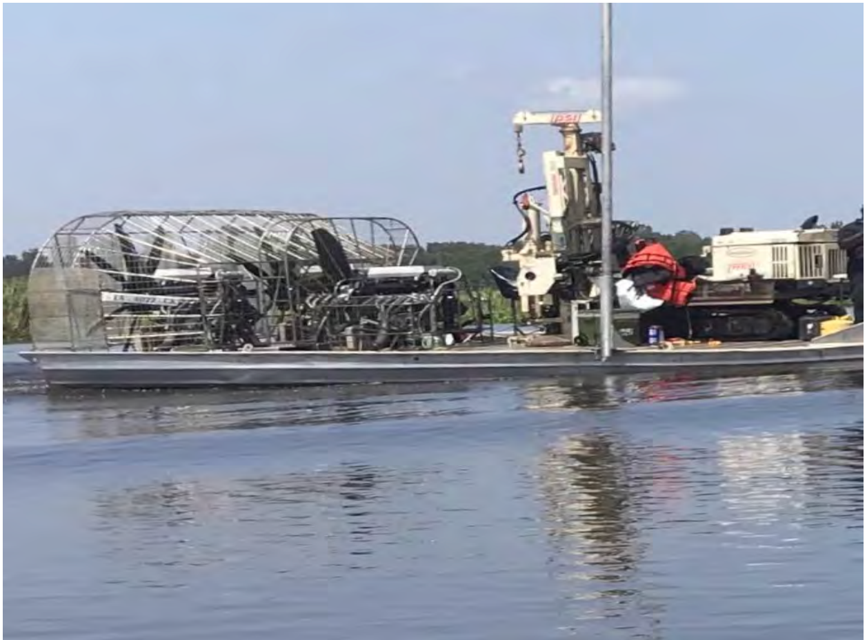
Figure.2: Airboat Mounted Drill rig
