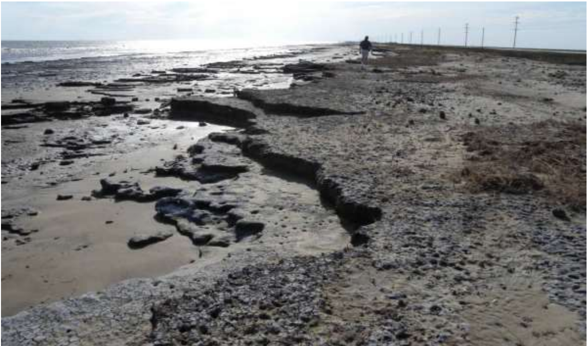
Figure 2A. Gulf of Mexico shoreline before construction of the Cameron Parish Shoreline Restoration Project (CS-0033); beach erosion had reached HW 82 at the southern margin of the Oyster Bayou project area.
