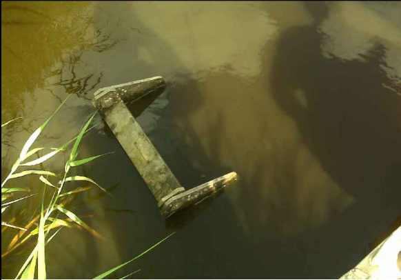
DEC PIPELINE CANAL PICTURE POINT 1
