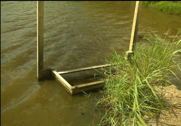
B1 CANAL PICTURE POINT 2
