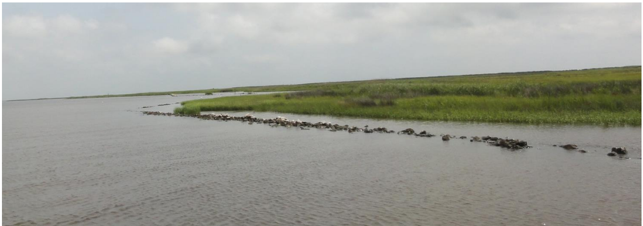
Photo No. 8 – Sabine Lake Foreshore Rock Dike, Low area of Rock
