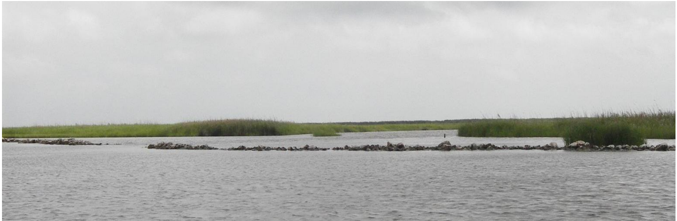
Photo No. 11 – Sabine Lake Foreshore Rock Dike, Low area at Willow Bayou bend (Same Location as Photo 10)
