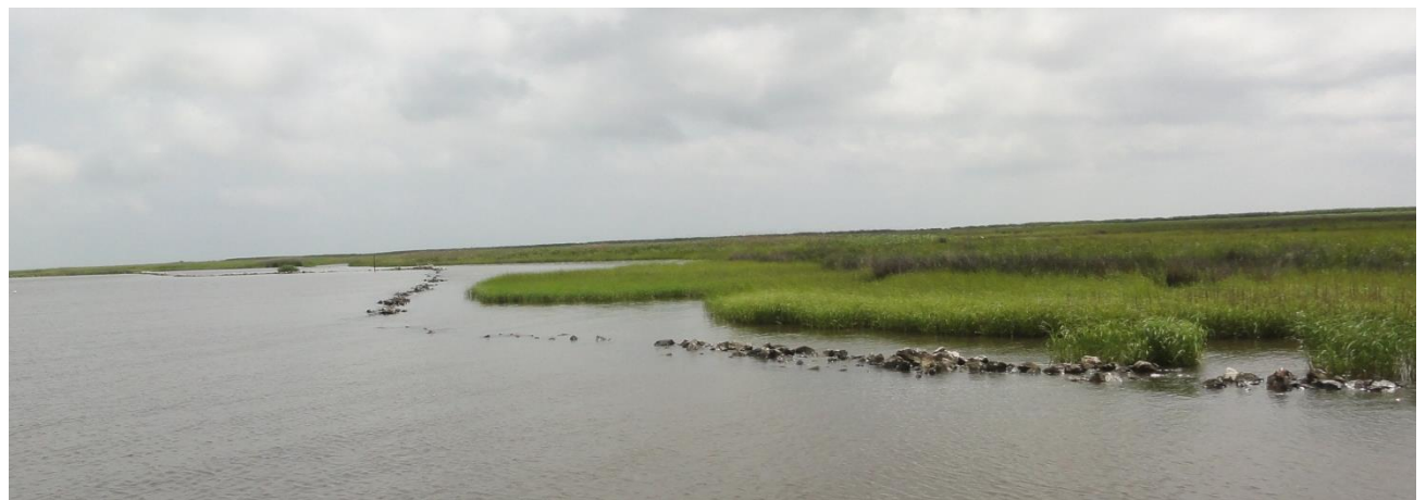
Photo No. 9 – Sabine Lake Foreshore Rock Dike, Low area of Rock
