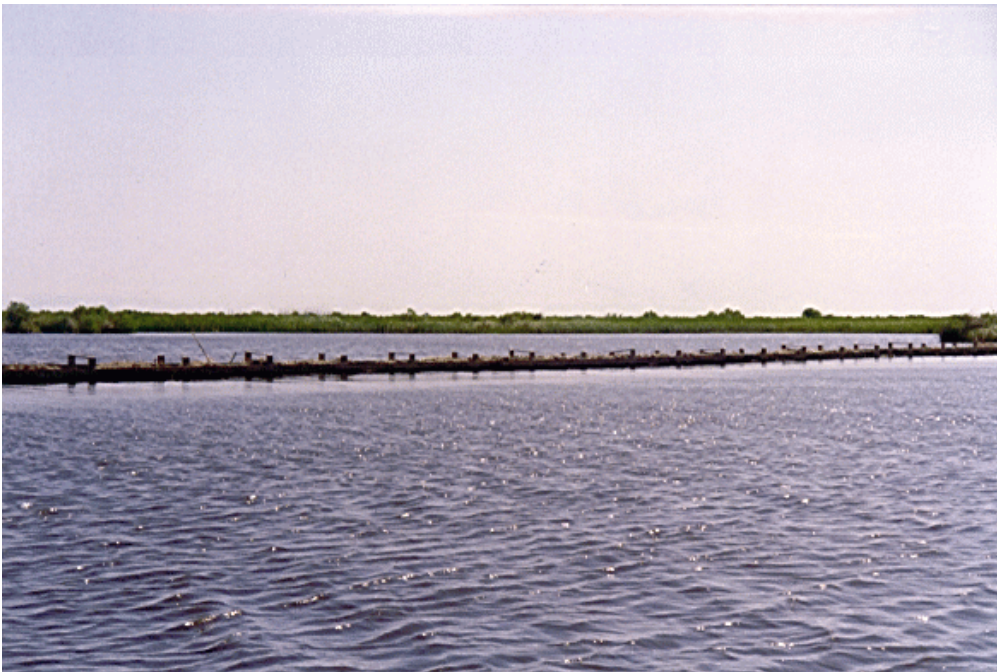
Figure A2. Group B hay bale fencing within the CS-19 project area showing wave damping ability and distance from shoreline the fences were constructed.
