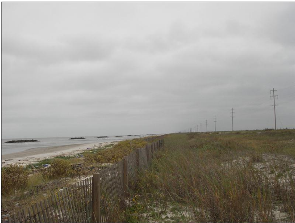
Photo No. 4, Typical sand fence section on easternmost end of project
