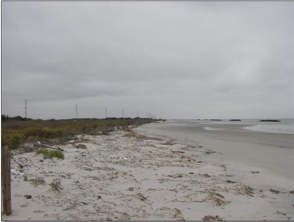
Photo No. 3, Long section of damaged fence
