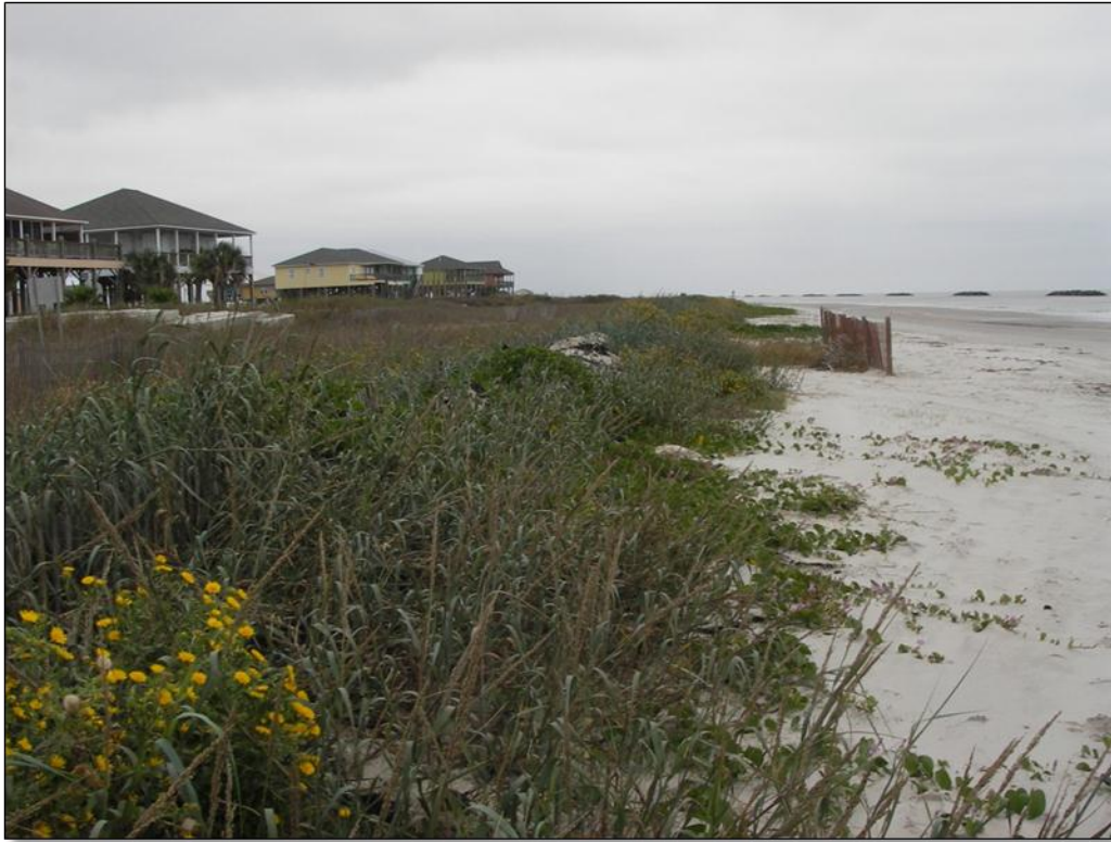
Photo No. 1 , Typical sand fence section on westernmost end of project
