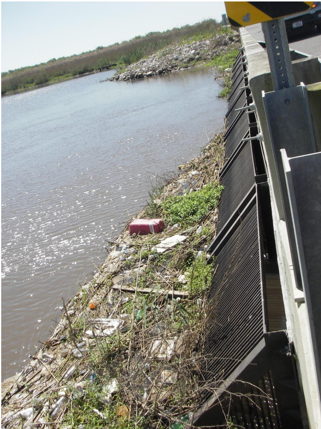
Photo No. 8, East Side of Box Culvert Structure (Looking South), Floating Debris
