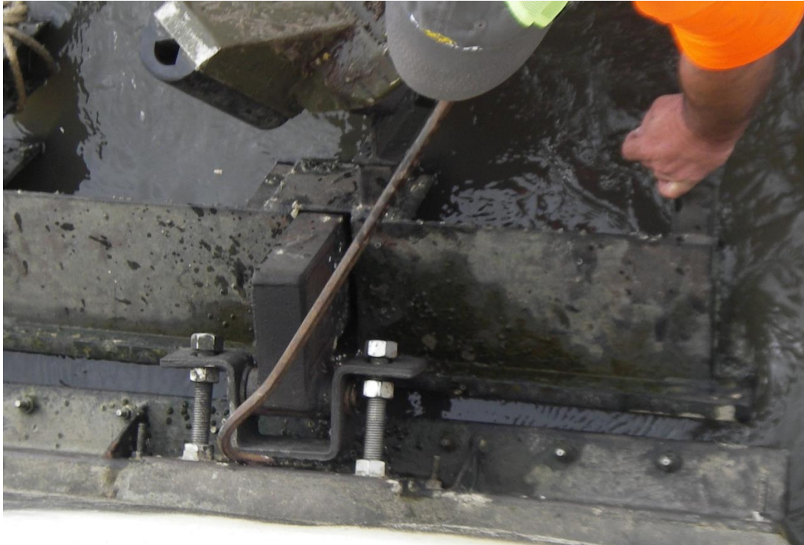
Photo No. 6, Anchor Rods on Flapgates, Nuts Loosening and Backing Off of Anchor Rod
