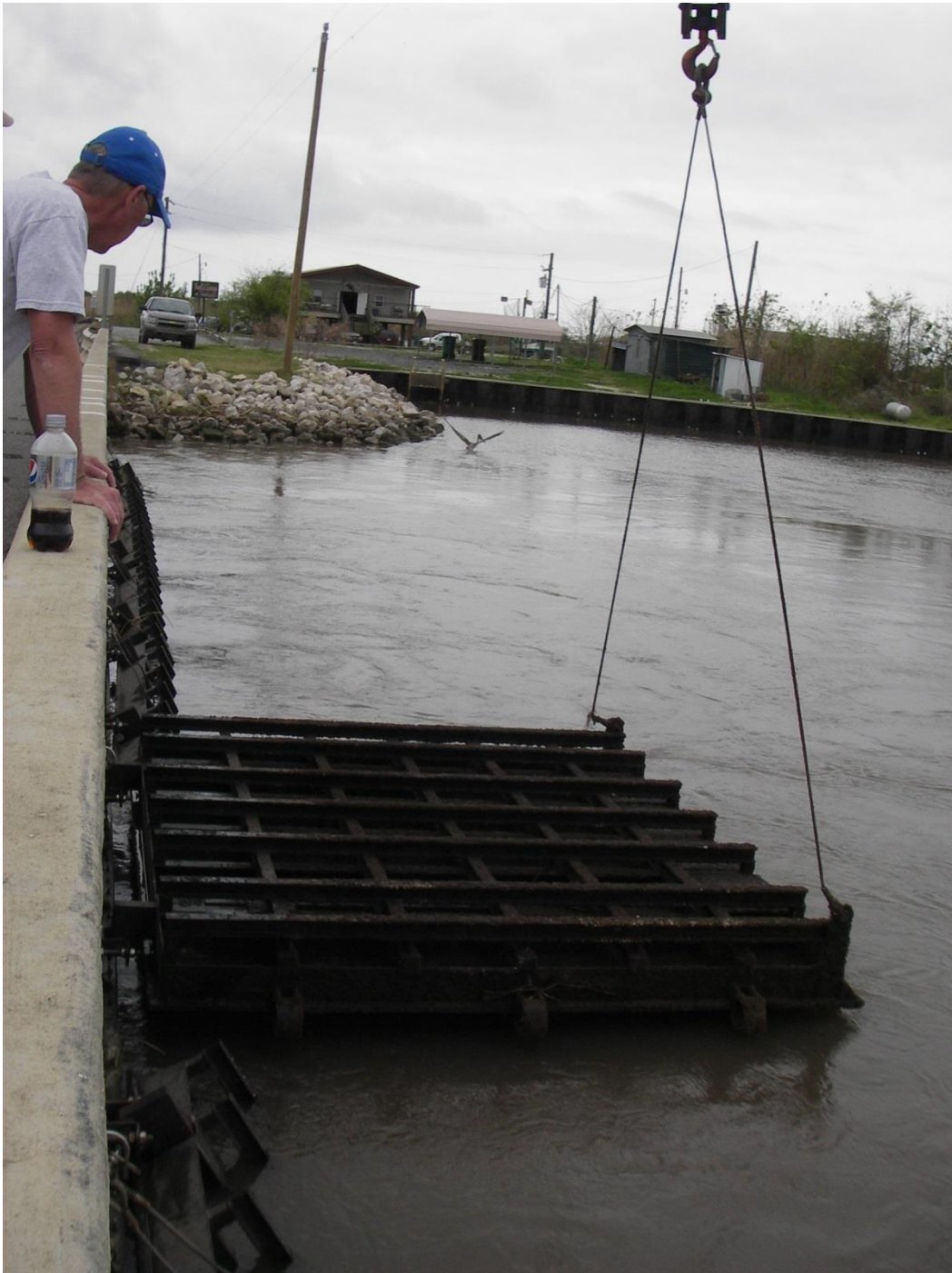
Photo No. 5, West Side of Box Culvert Structure, Flap Gate, Rock Armoring, & Steel Bulkhead
