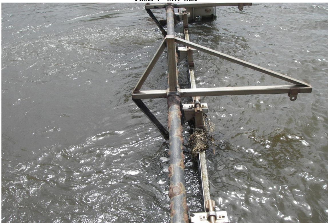
Photo 5—pillow block on SRT Gate flap & railing rust
