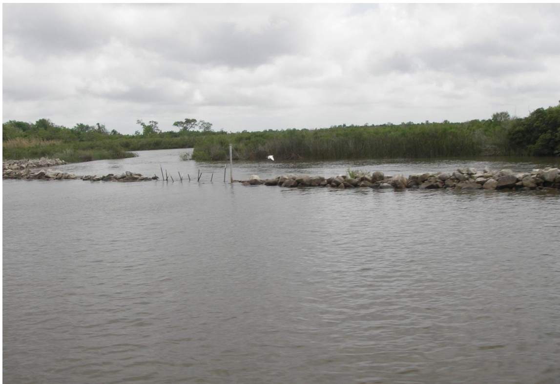
Photo 12 —gap in dike and break near closure behind dike
