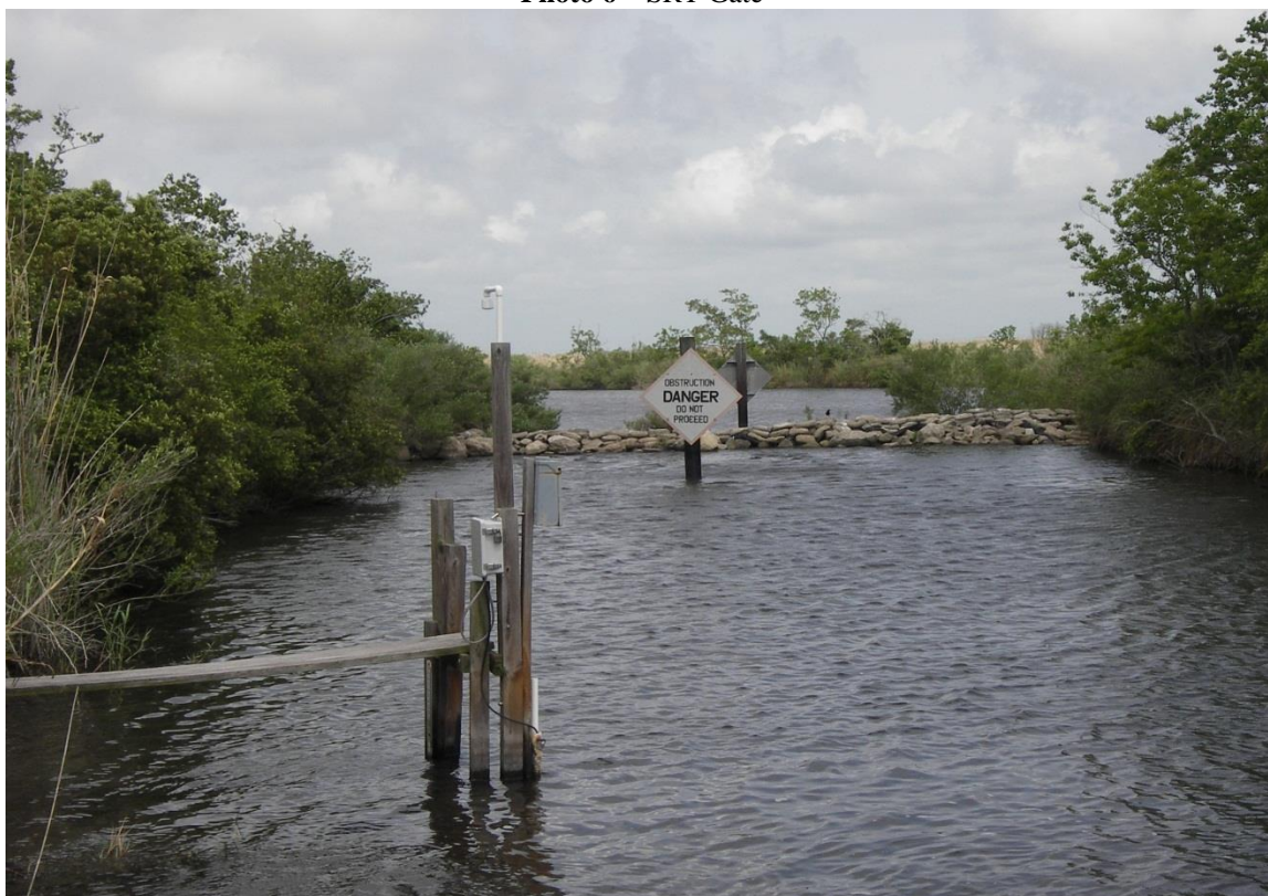
Photo 7—Rock plug near SRT Gate
