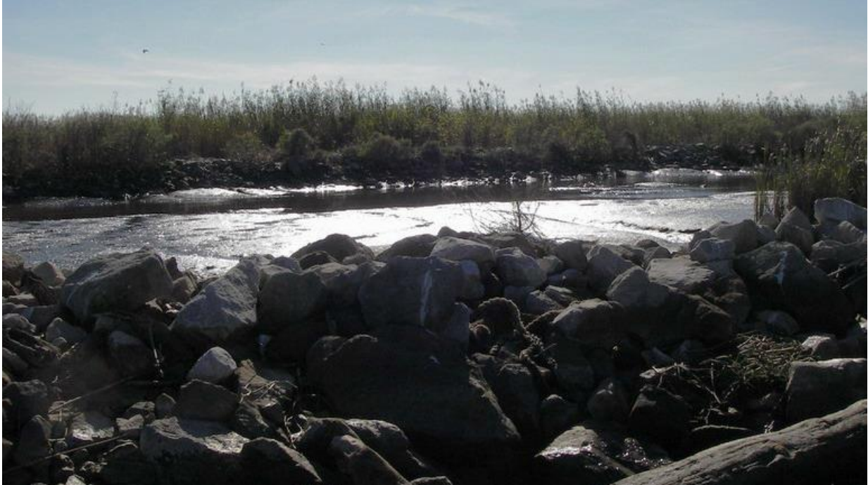
Figure 12. Sedimentation and vegetative growth between the GIWW rock dike and dredge material levee along the north side of the impoundment.
