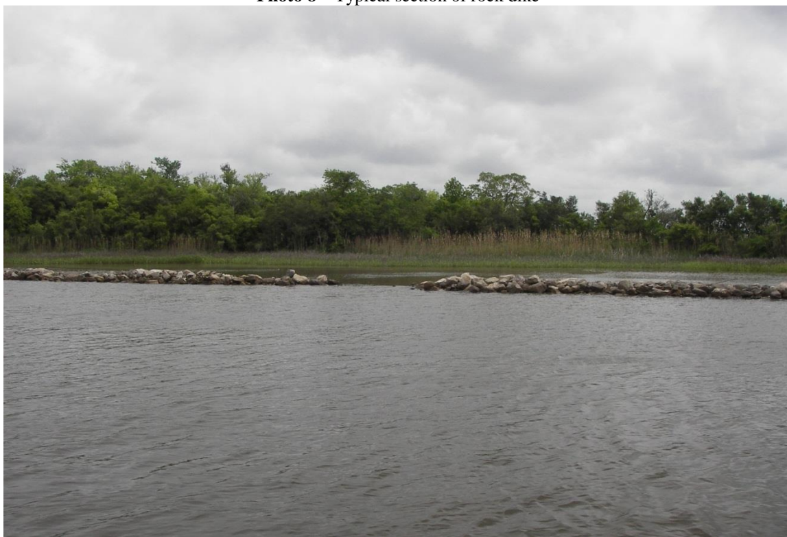
Photo 9 —gap in dike with new vegetation between dike & shoreline
