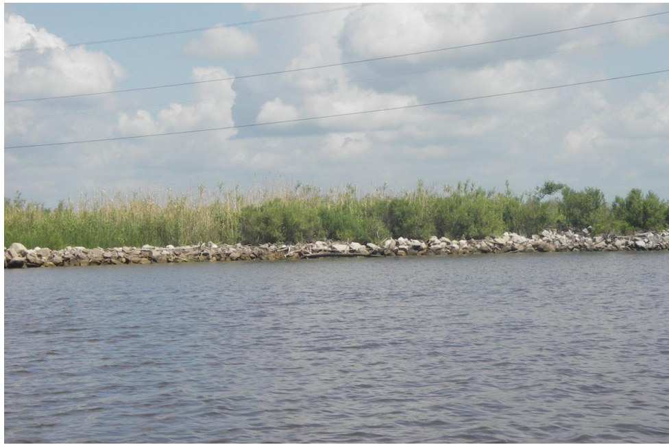
Photo No.1, Typical Rock Dike
