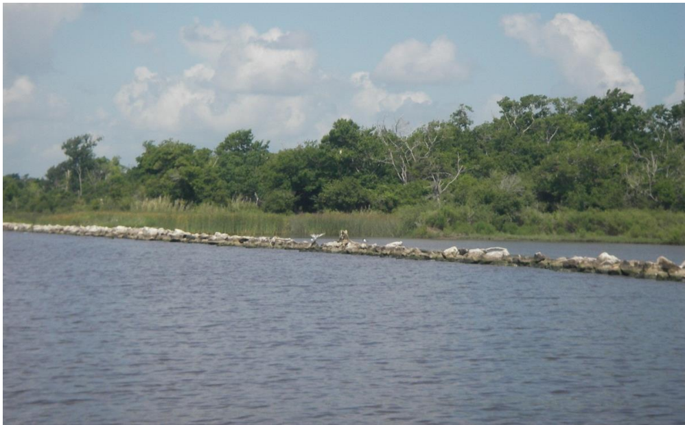
Photo No.2, Accretion behind Rock Dike
