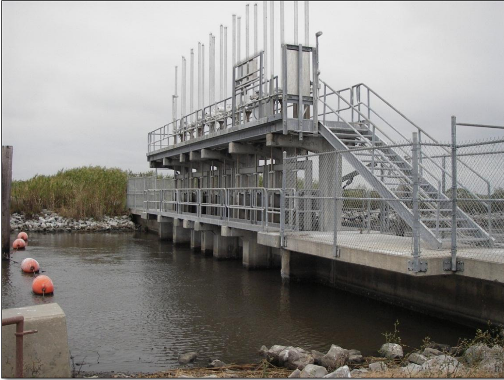
Photo No. 1 , Hog Island Gully Structure looking from the Hwy 27 side
