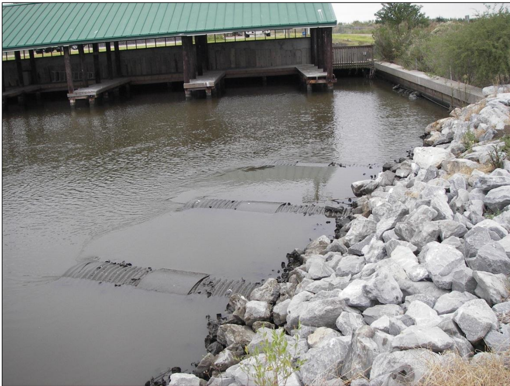
Photo No. 4, Headquarters Structure marsh side culverts with riprap
