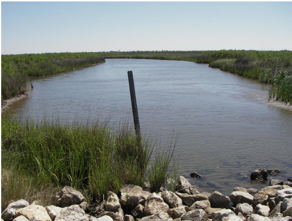
Photo No. 8, Structure No. 8, Rock Plug - Vegetation on Project Interior (April 2014)
