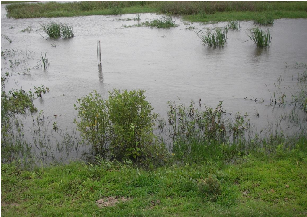
Photo No. 1, Structure No.1, Outlet Side
