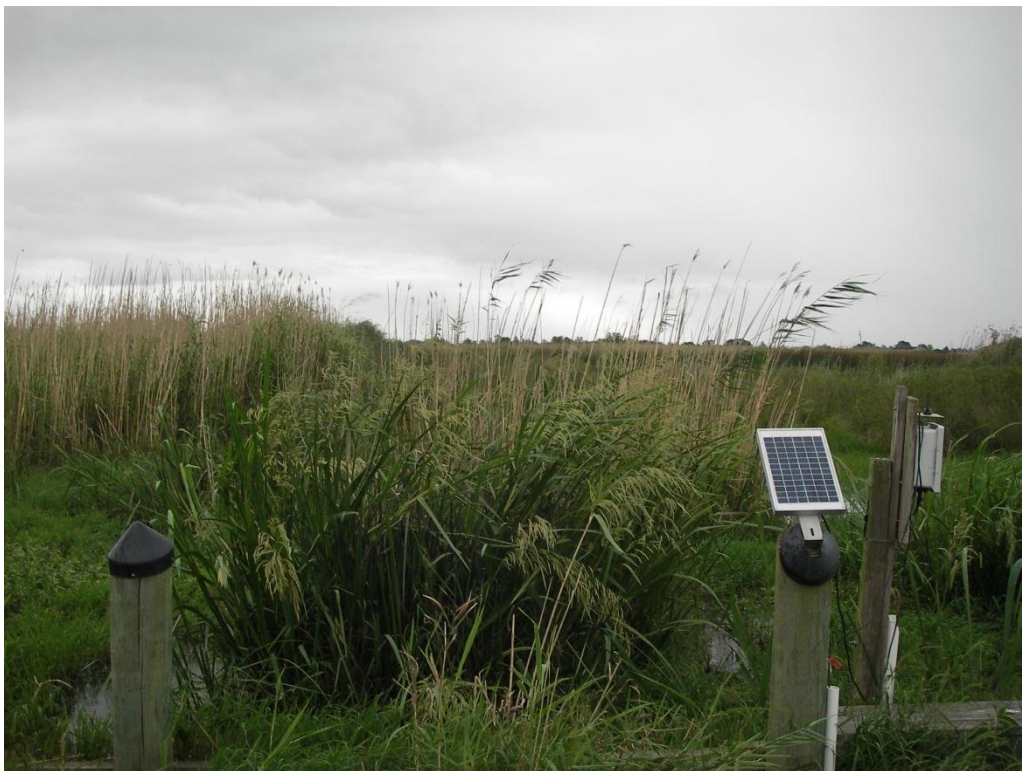
Photo No. 4 , Vegetation in Inlet Channel to Structure No.1
