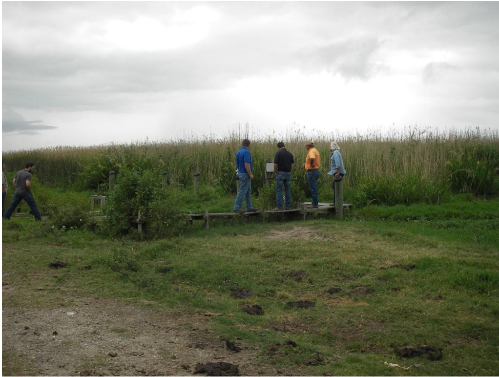
Photo No.3 , Structure No.1, Walkway Looking Northwest – Vegetation in Channel
