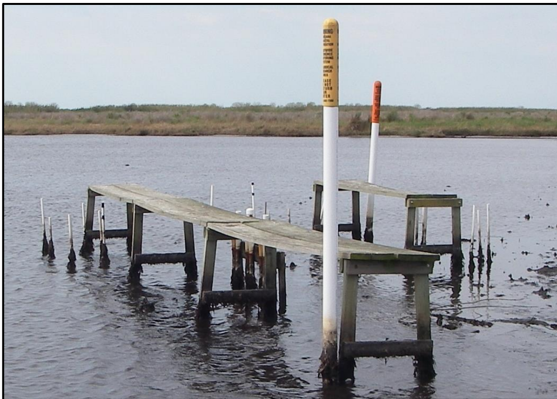
Figure 2.5b. Photograph of a boardwalk in a marsh that washed away. The portion of the teeth that is normally beneath the surface is exposed.
