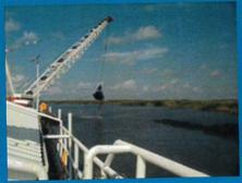
Digging access—spoil being placed on the landward side of the dike to be constructed
