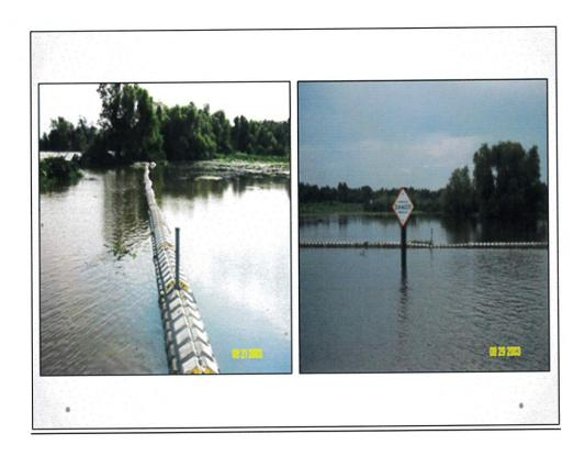
Approximately 1,857 ft (566 m) of parallel straight-walled fiberglass sheet pile divided among three replicate treatment blowouts (V1, V2, V3).
