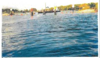
Weirs constructed with a boat bay aid in the effective management of hydrology while still allowing the passage of small boats and vessels.
