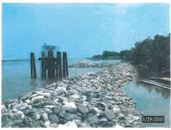
Where existing structures were encountered, such as the crossing of the freshwater delivery system to Grand Isle pictured above, the alignment of the structure was altered.
