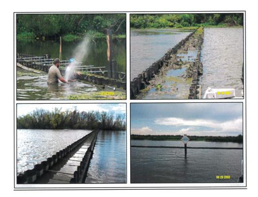
Approximately 1,283 ft (391 m) of 24 inch (0.61 m) high A-Jacks concrete blocks in an interlocking double row with two staggered rows of Zizaniopsis miliacea (Michx.) Doell & Aschers. planted on five foot centers between it and the shoreline divided among three replicate off-bank treatments (J1, J2, J3).
