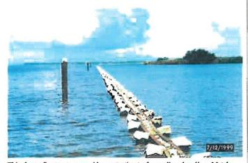
This sheet-pile structure provides protection to the eroding shoreline. Metal caps were placed on the pilings to prevent the rotting of the wood.
