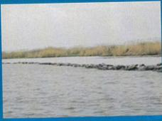
Constructed dike with what's left of the spoil behind it. Dike has already begun to settle which was expected.
