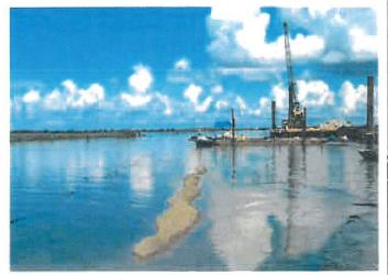
In order to prevent the heavy rock riprap from settling too deep in the organic soil, geo-textile cloth was first put down and used as a base.
