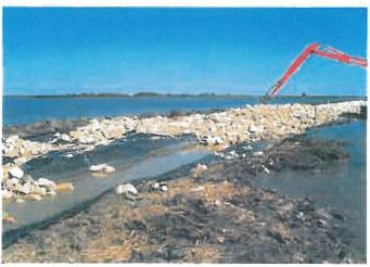
The narrow, eroding shoreline of Bayou DeCade was reinforced with rock in order to help restore the hydrology of the Brady Canal area.
