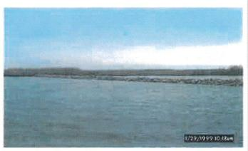
Rock riprap which can withstand the destructive forces of wave energy helps to maintain the integrity of the shoreline.
