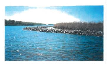
Limestone riprap was placed within a 4.3 mile reach along the north bank of the GIWW between the Vinton Drainage Canal and Perry Ridge.
