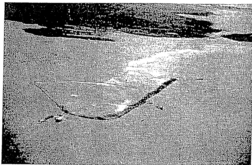
Marsh lobe under construction at Big Island.
