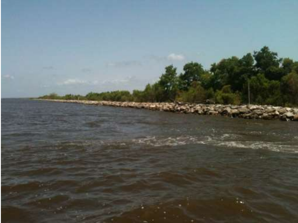
Photo #1 – Shoreline Protection
