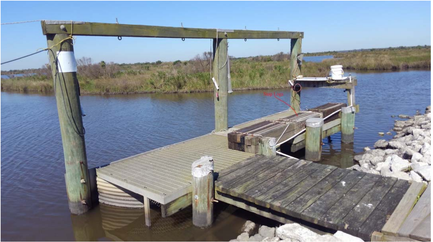
Photo #3 – Water Control Structure (Culverts Submerged)
