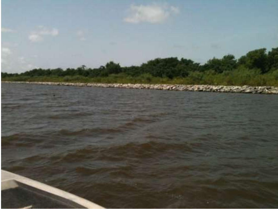
Photo #1 – Shoreline Protection
