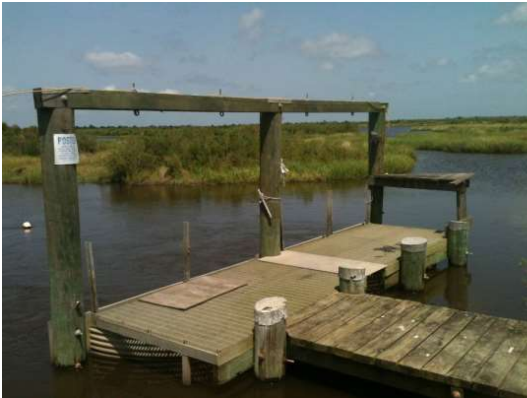
Photo #2 – Water Control Structure
