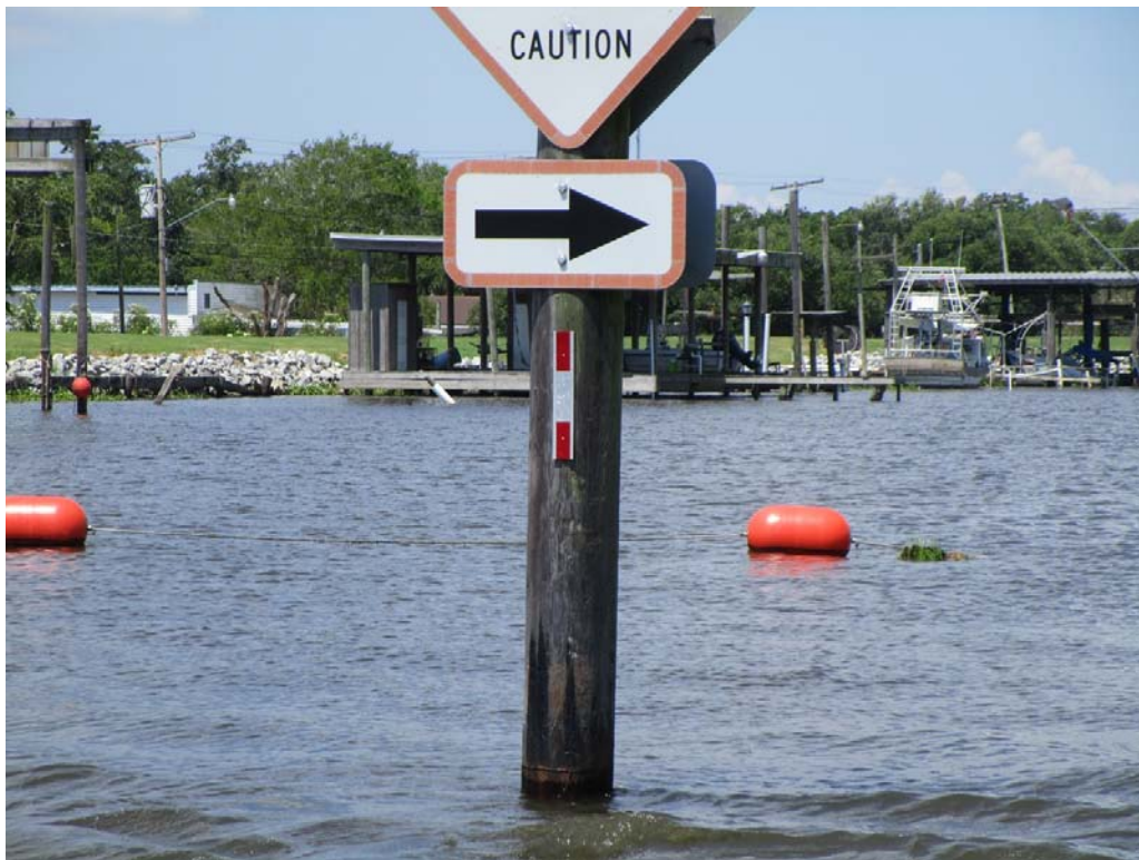
Photo #4 – New reflective tape on piles (Goose Bayou)
