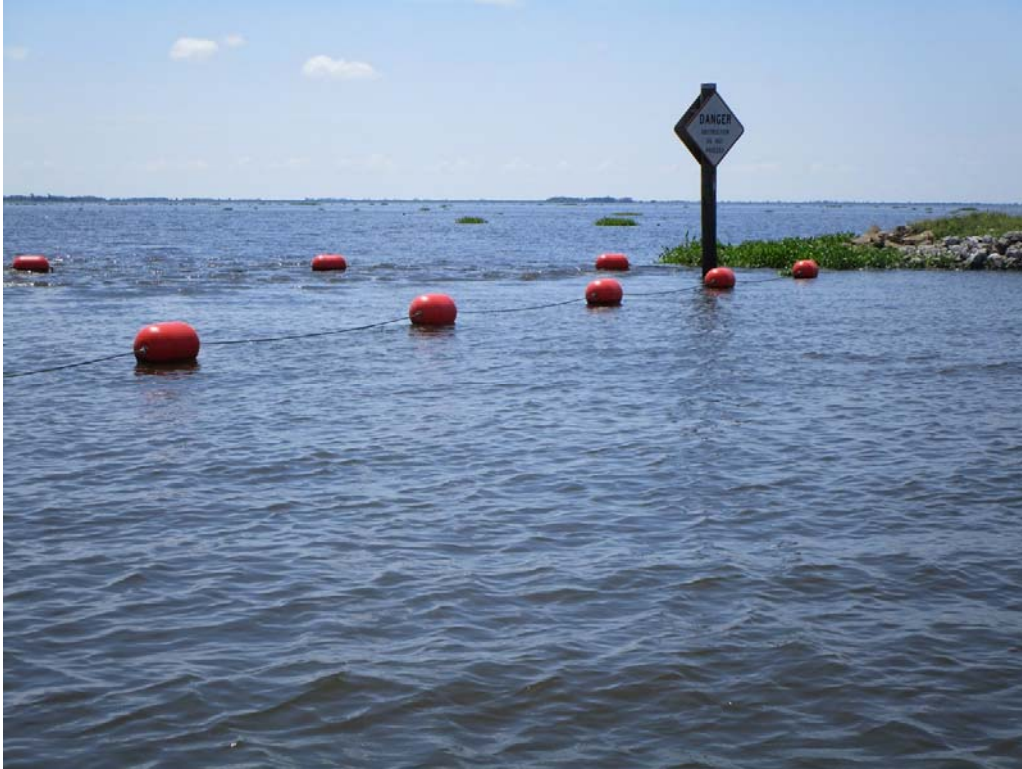
Photo #3 – New barrier floats and cables (Goose Bayou)
