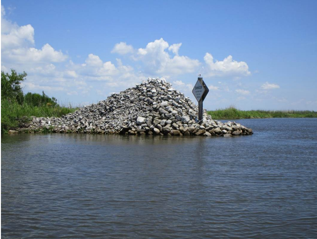
Photo #1 – Riprap stockpile for weir restoration (Bayou Dupont)
