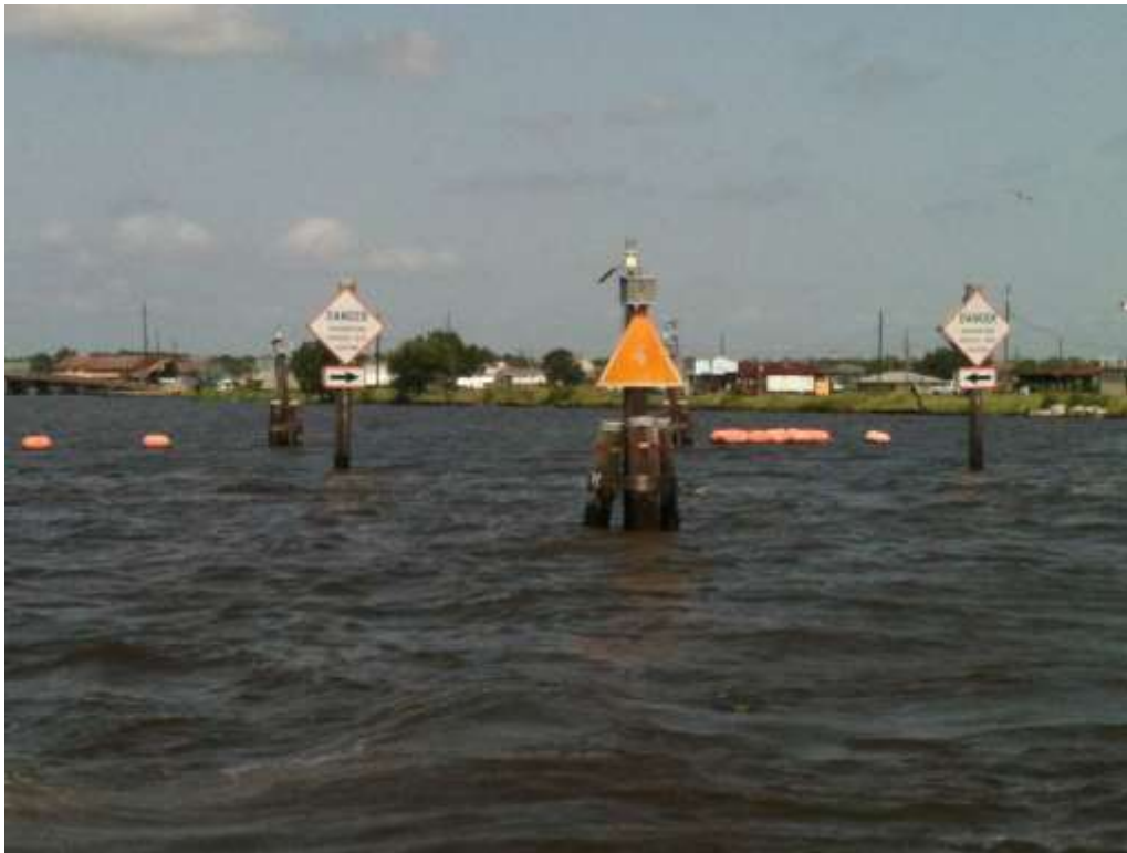
Photo #2 – Goose Bayou Pile Cluster
