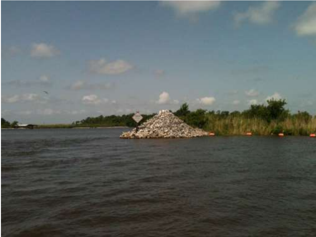
Photo #1 – Bayou Dupont Canal Weir
