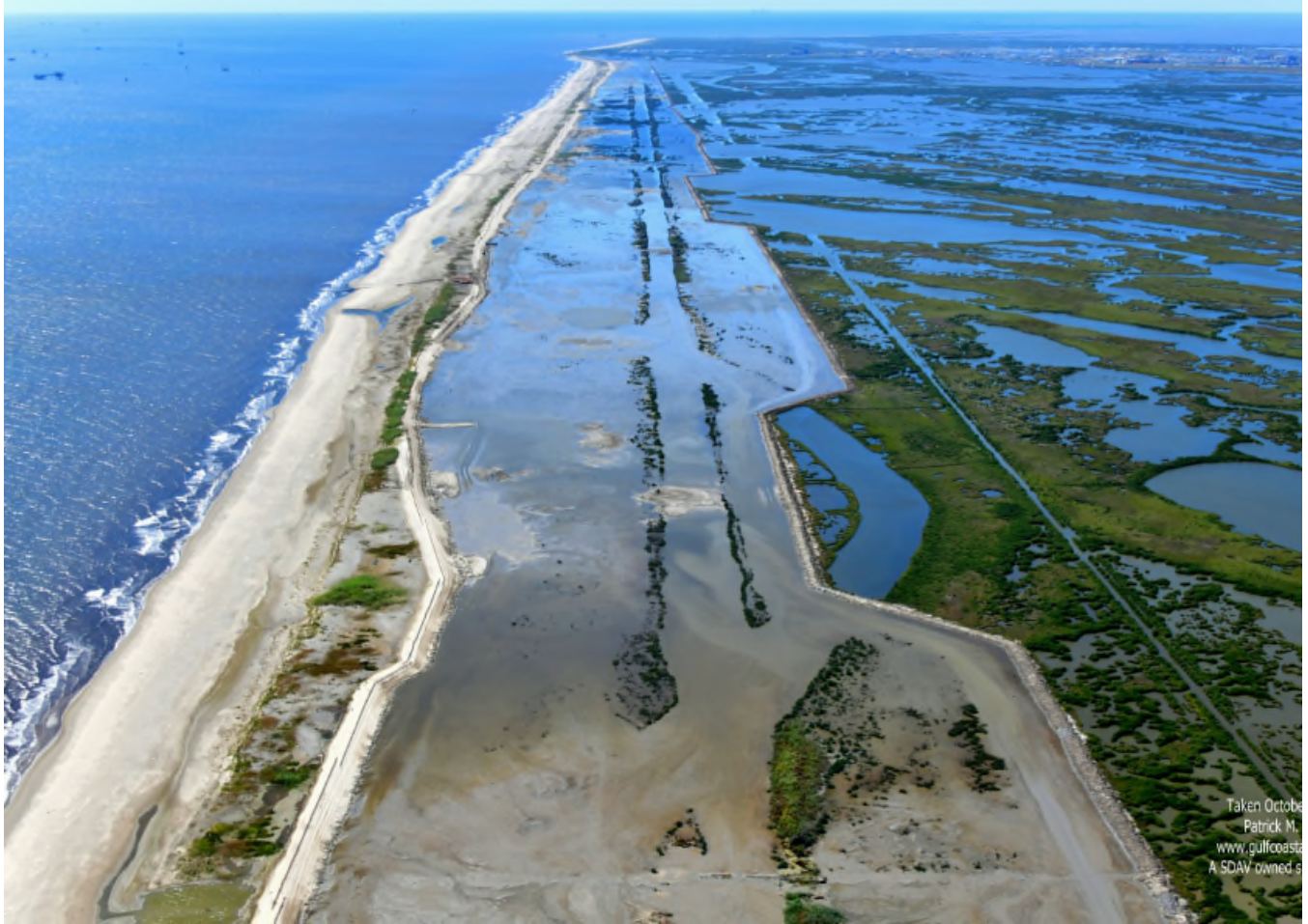
Figure 14: MCA Increment 3 Looking West Post Fill Operation (Still Dewatering)
