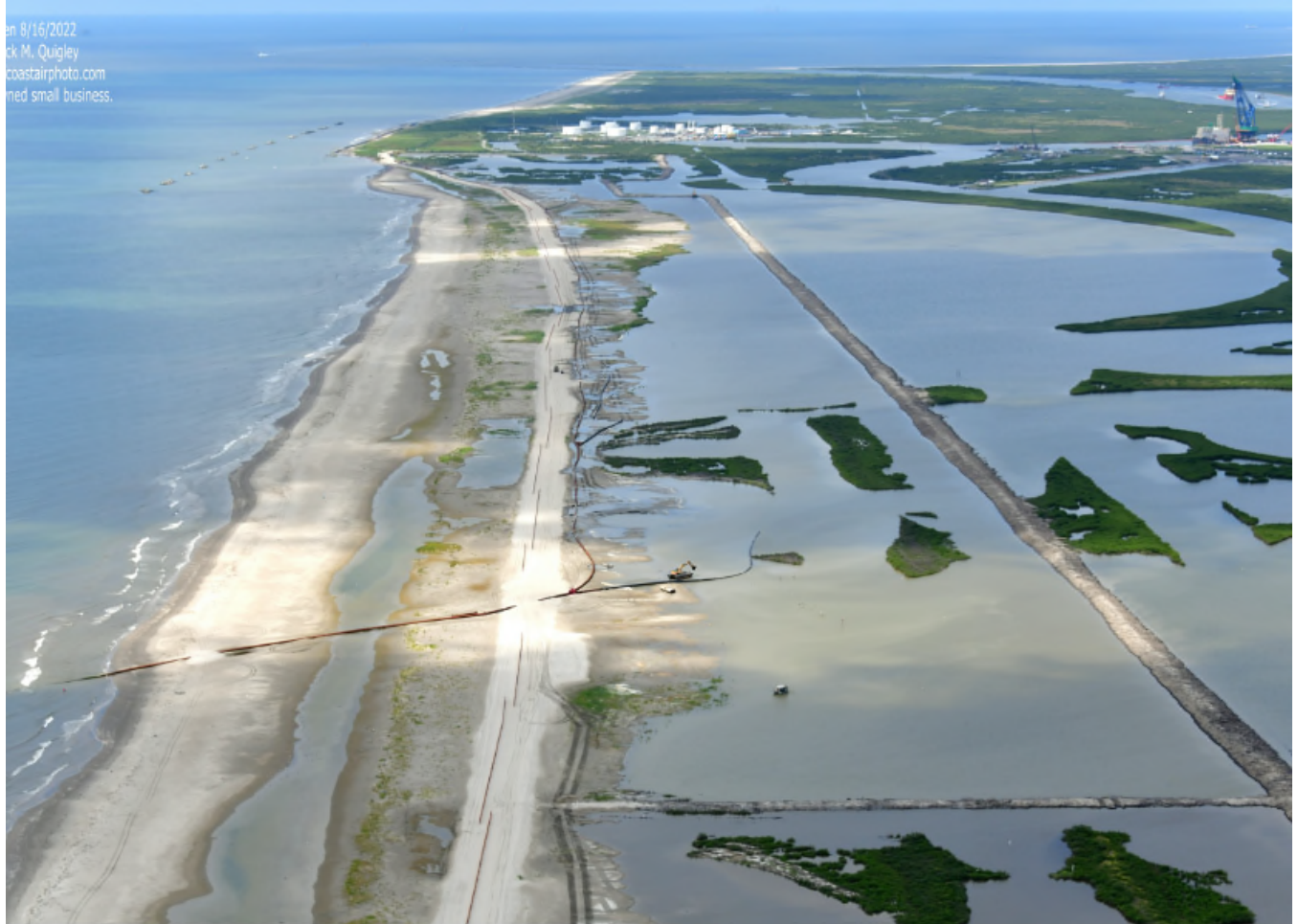
Figure 9: MCA Increment 1 Looking West During Fill Operation
