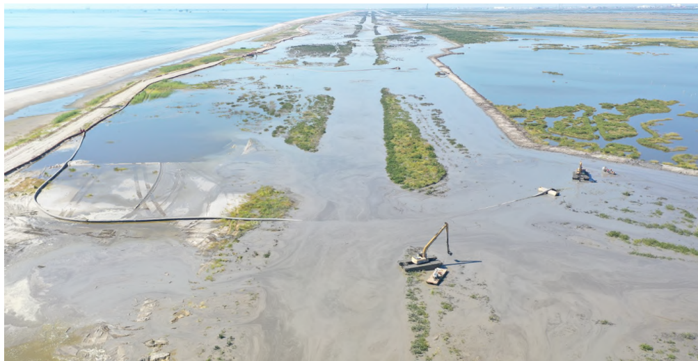
Figure 7: Hydraulic Fill Placement Increment 3 Looking West
