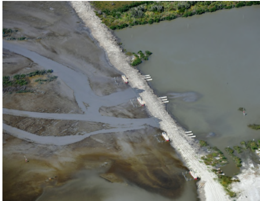
Figure 8: Dewatering Weirs at Eastern Limit of Increment 4
