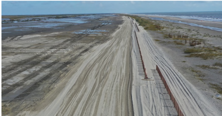
Figure 6: Sand Dune Reconstruction and Sand Fence Installation
