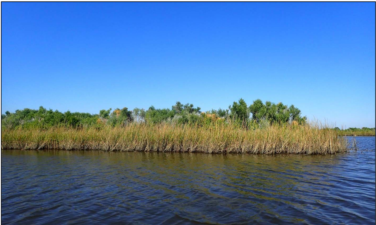
Photo 4. Terrace 8, showing shrubs growing on the crown and expanding, planted Spartina alterniflora growing along the base of the slope.
