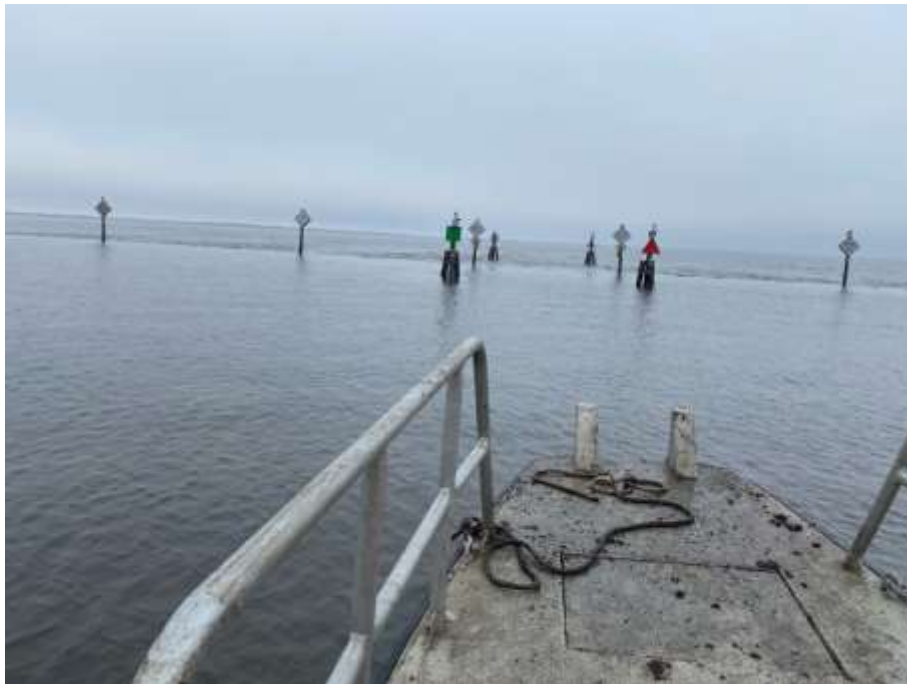
Photo 2. Goose Bayou Canal weir, looking east. The weir has settled below the waterline.
