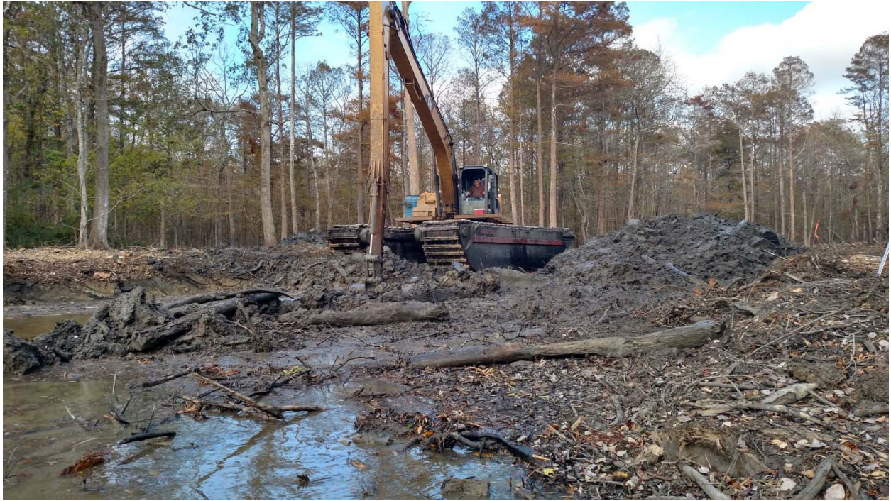
Photograph 5 - Long Reach Excavator excavating spoil while encountering submerged logs.
