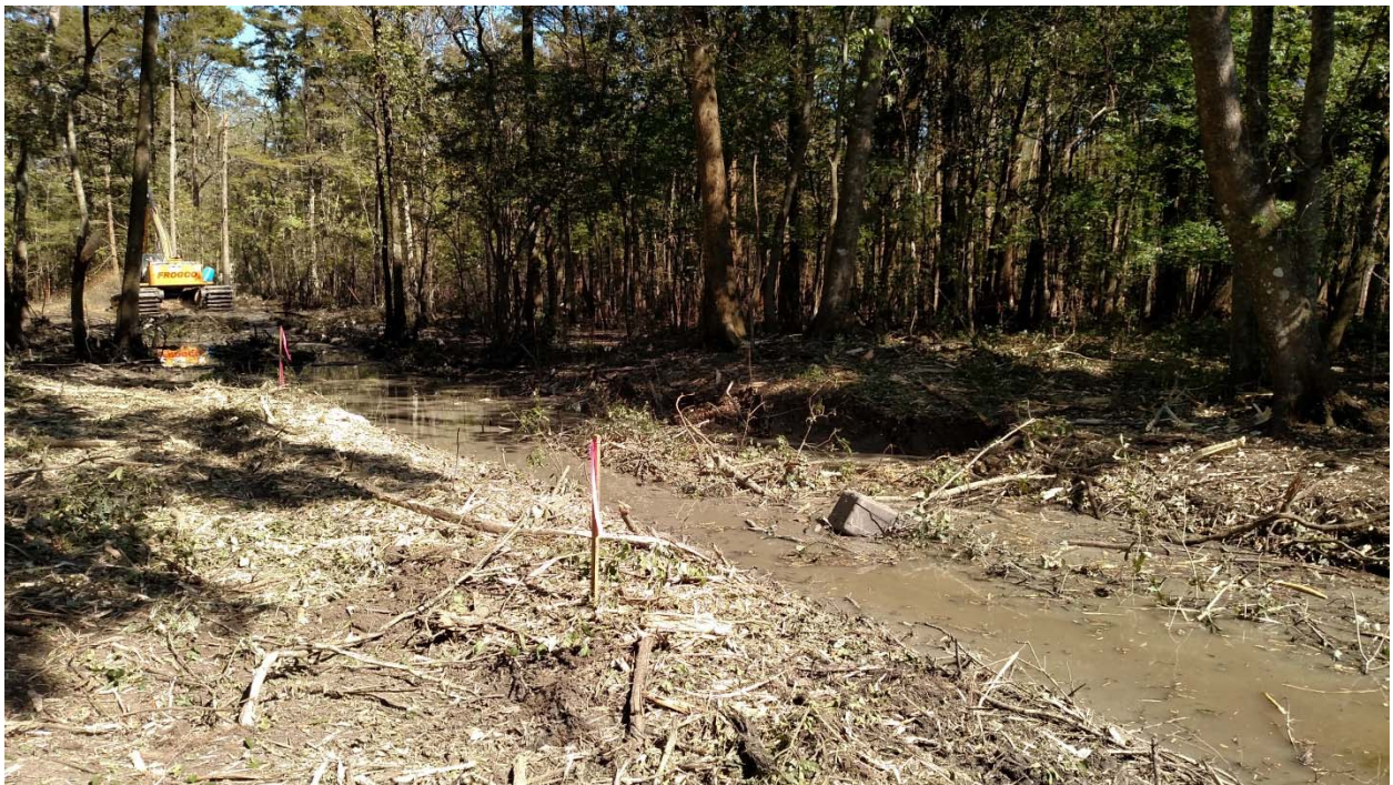
Photograph 2 - Contractor clears a path to backside of gap and then works back to front.
