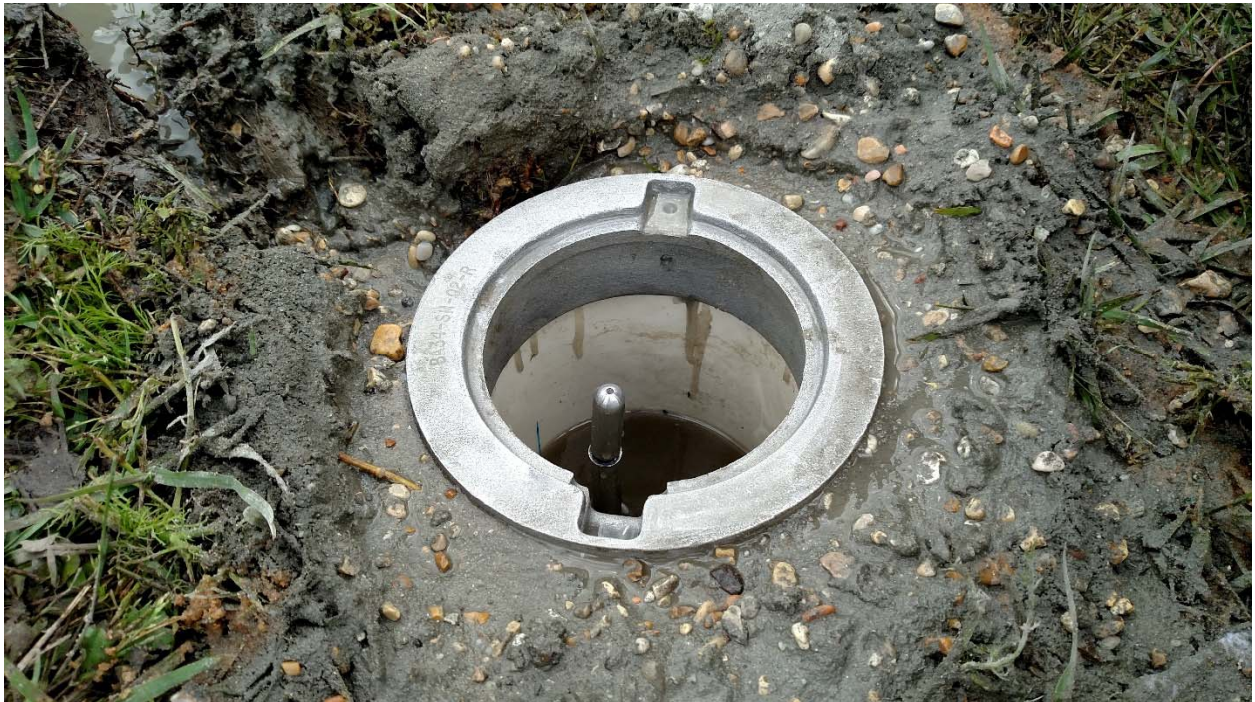
Photograph 22 – Bullet cap screwed onto the last rod with concrete drying around the PVC shell.
