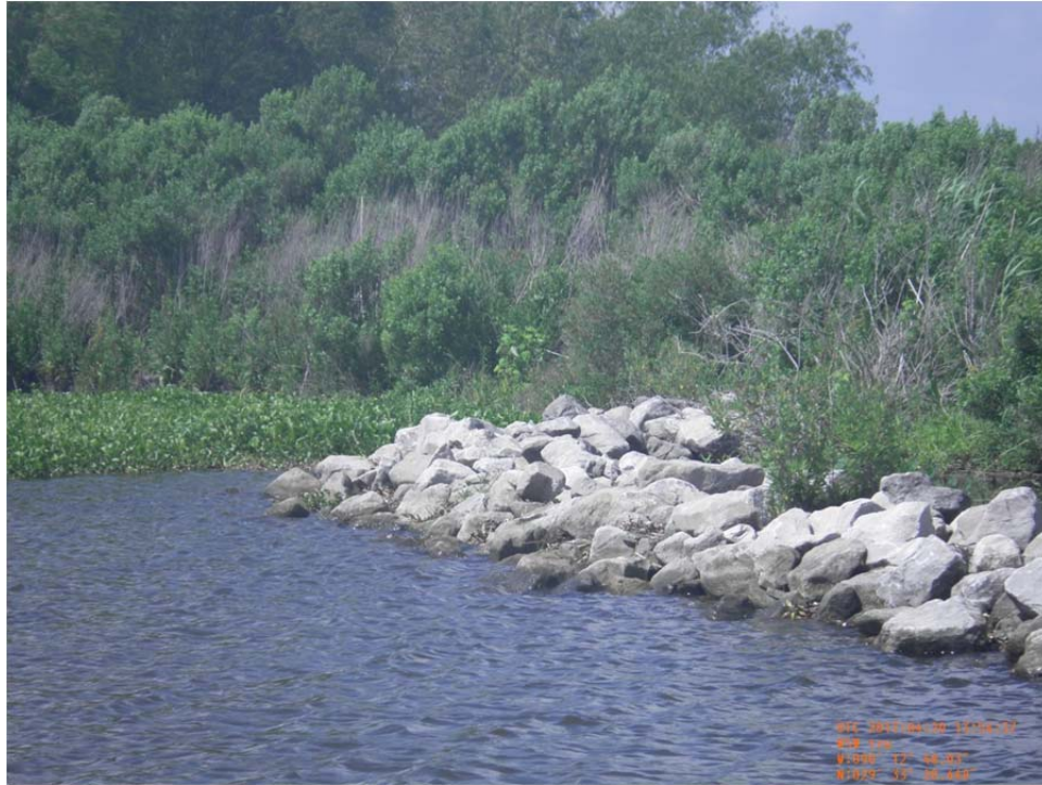
Photo No. 15 – view of rock revetment (CU#2- West Site) tie-in along existing channel near Sta. 26+47.
