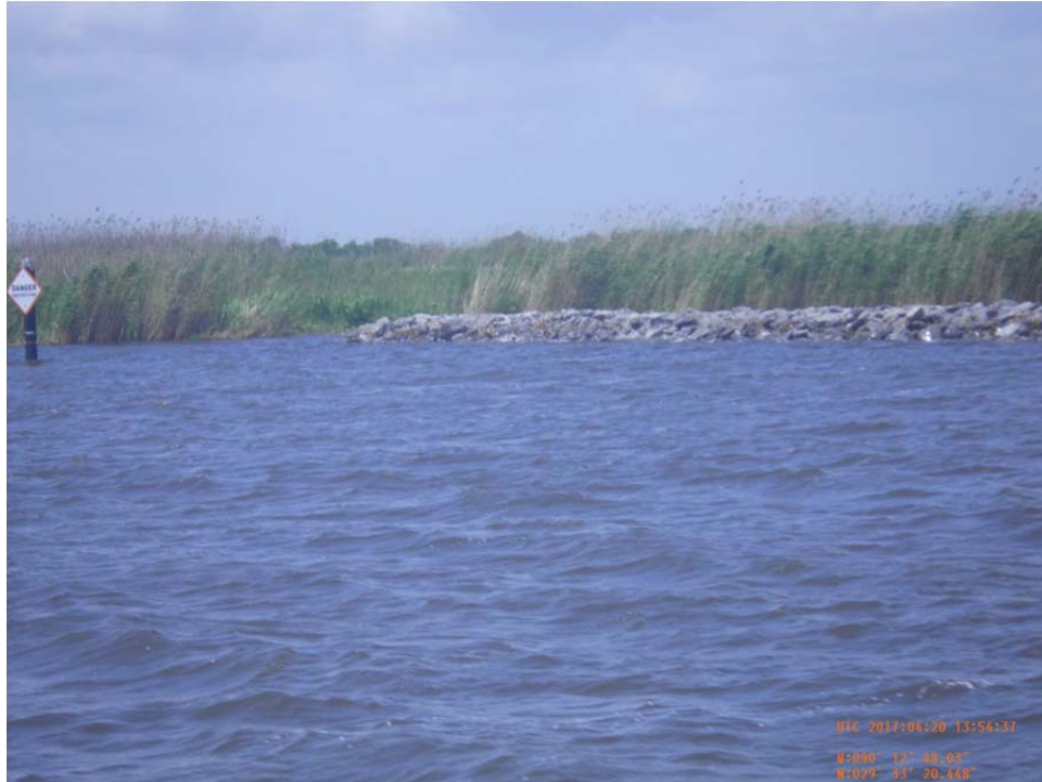
Photo No. 48 – view of rock revetment to bank tie-in at the south end (Sta. 0+00) of CU #7 & 8 (Revetment #6) along the west bank of Bayou Perot.
