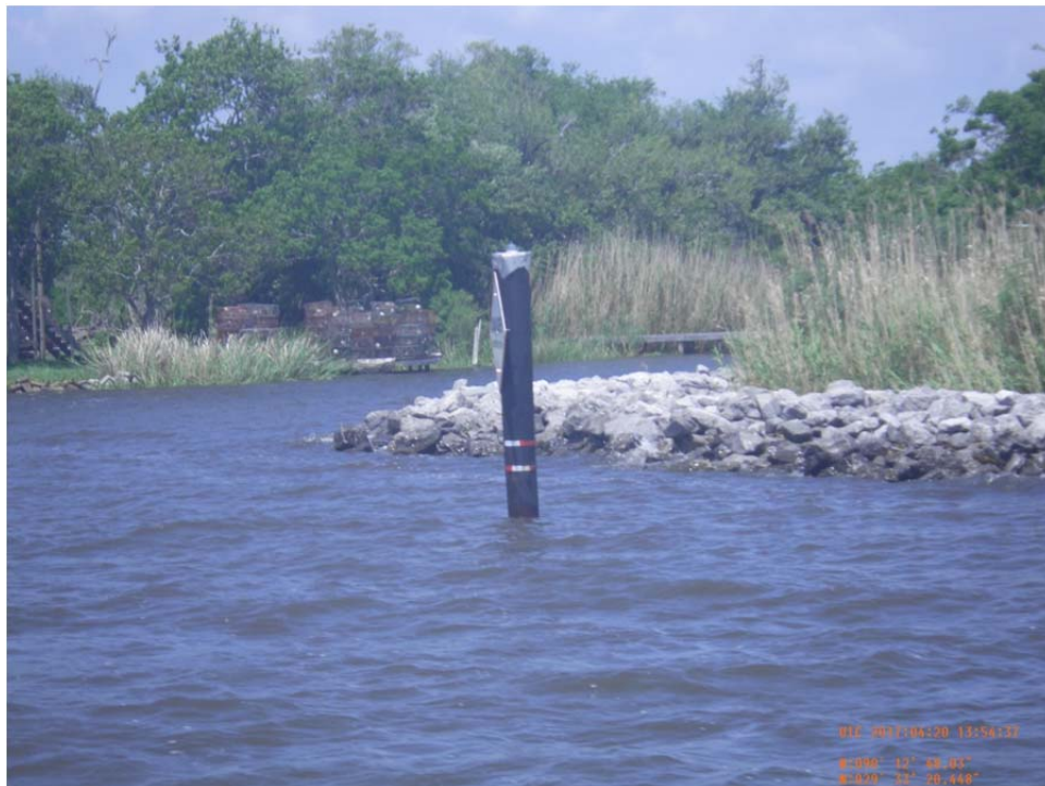
Photo No. 63 - view of rock revetment tie-in to bank at the western end of CU # 7&8 (Revetment #1) near Sta. 0+00.
