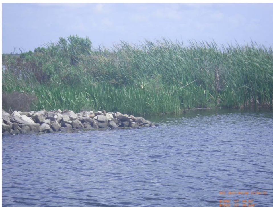
Photo No.32 – view Rock Revetment (CU#6) at the far southern end that ties into the bank of an existing oilfield canal near Sta. 305+00.
