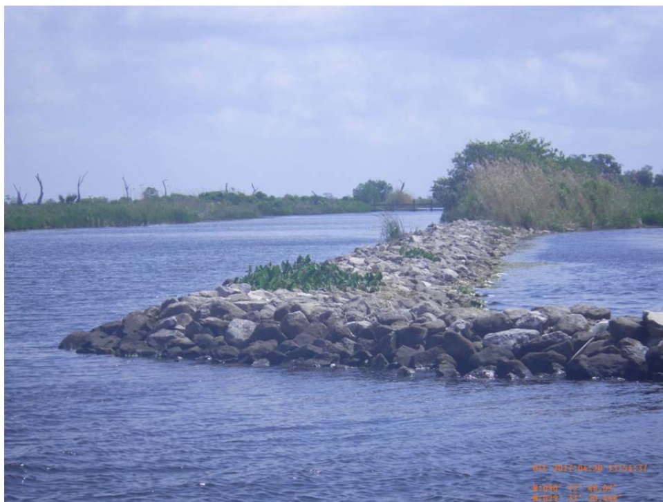
Photo No. 31 – view of CU#4 (Reach 1) rock dike along existing canal along east bank of Bayou Rigolettes that ties into the Concrete Wall near 4+50.
