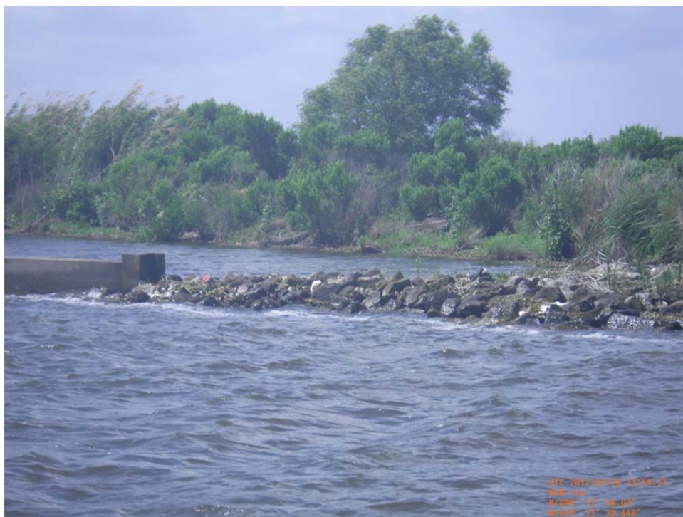
Photo No. 21 – view of rock revetment to concrete wall tie-in at Sta. 36+83 of CU#2 (East Site).
