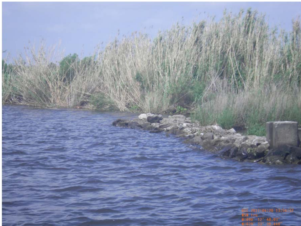
Photo No.24 – view of the rock tie-in from concrete wall to bank of CU#4 (Reach 2) along the west bank of the Harvey Cutoff Canal near Sta. 0+00.
