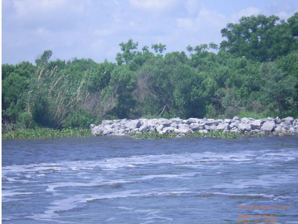
Photo No. 52 - view of rock revetment tie-in to bank at south end of CU # 7&8 (Revetment #3) near Sta. 0+00.
