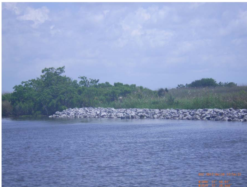
Photo No. 60 - view of rock revetment tie-in to bank at southern end of CU # 7&8 (Revetment #2) near Sta. 0+00.
