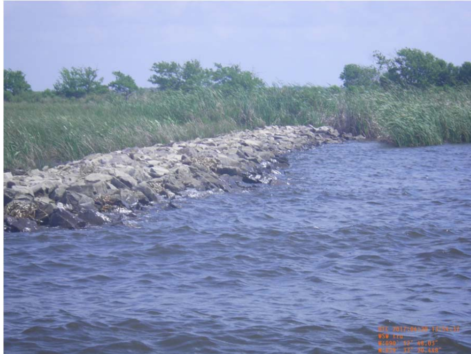
Photo No.1 – view of rock revetment to bank tie-in on southern end of CU#3 near Sta. 108+65.
