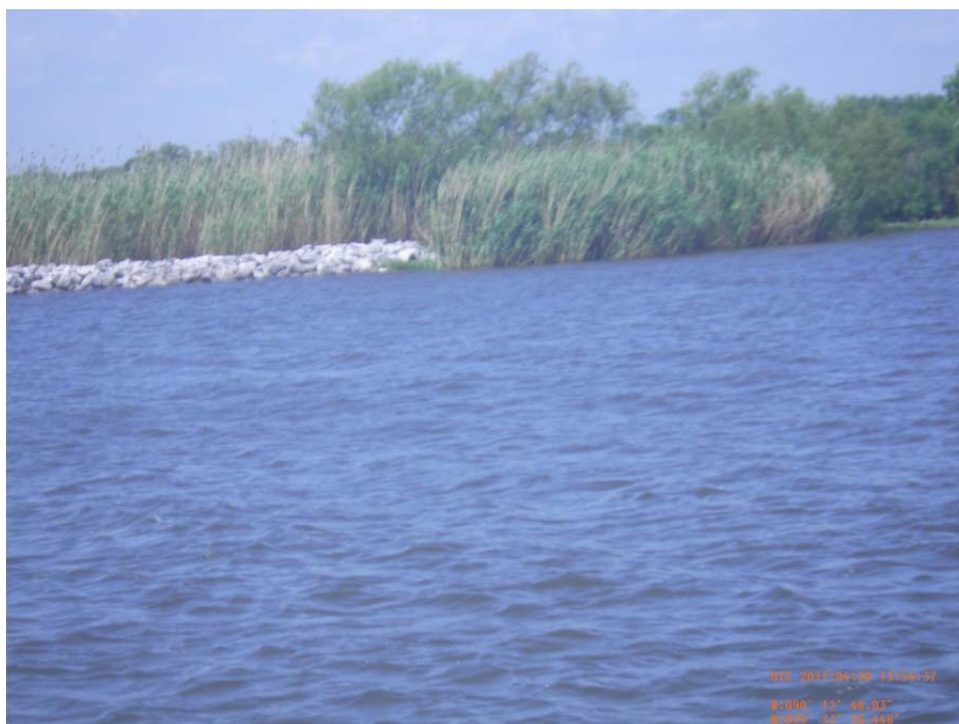
Photo No. 61 - view of rock revetment tie-in to bank at eastern end of CU # 7&8 (Revetment #1) near Sta. 64+64.
