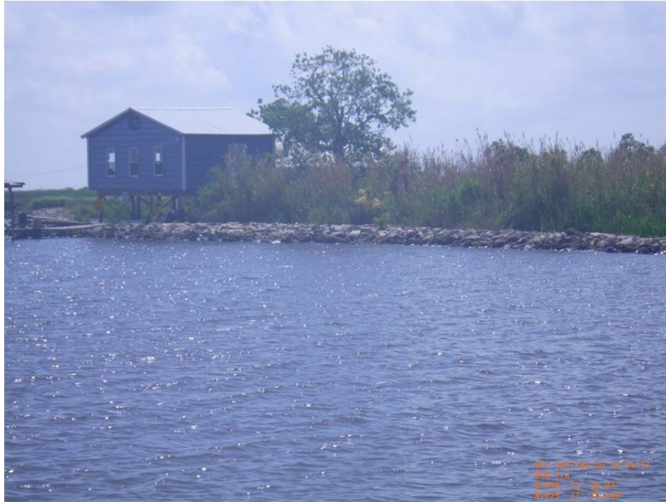
Photo No.5 – view of rock revetment (CU#3) along south shoreline of Bayou Perot at the entrance to Little Lake near an existing camp location at Sta. 3+00.
