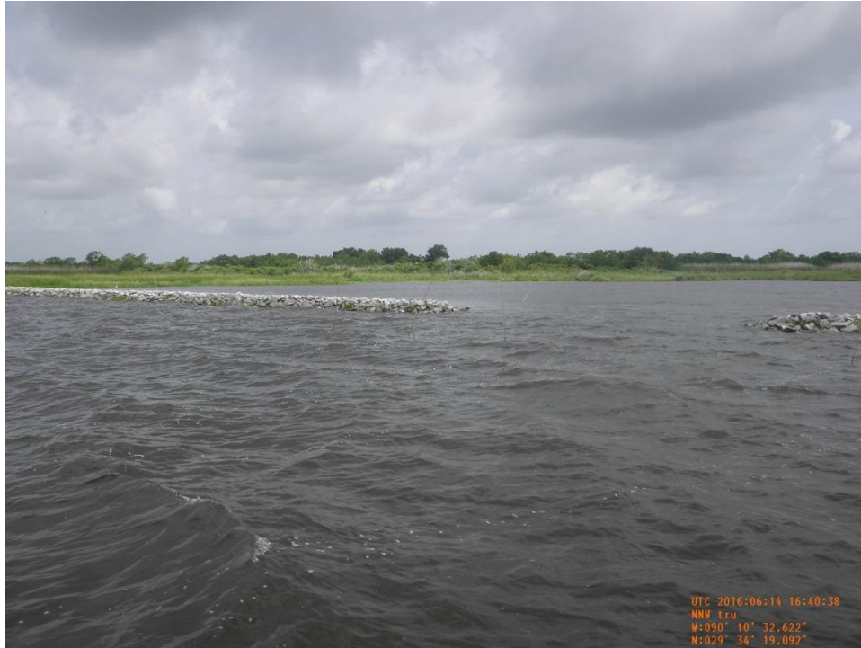
Photo 55: CU#8 fish dip on Revetment 1 near Sta. 53+00.
