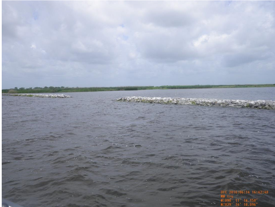
Photo 57: CU#8 fish dip on Revetment 1 near Sta. 11+00.
