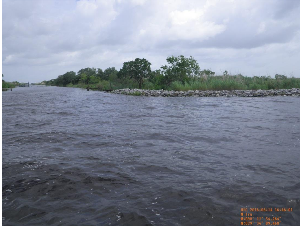
Photo 59: CU#8 Rock Dike bank tie-in near Sta. 0+00.
