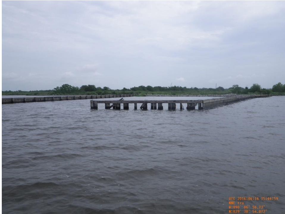
Photo 43: CU#6 rock revetment tie-in to timber bulkhead near Sta. 201+00.
