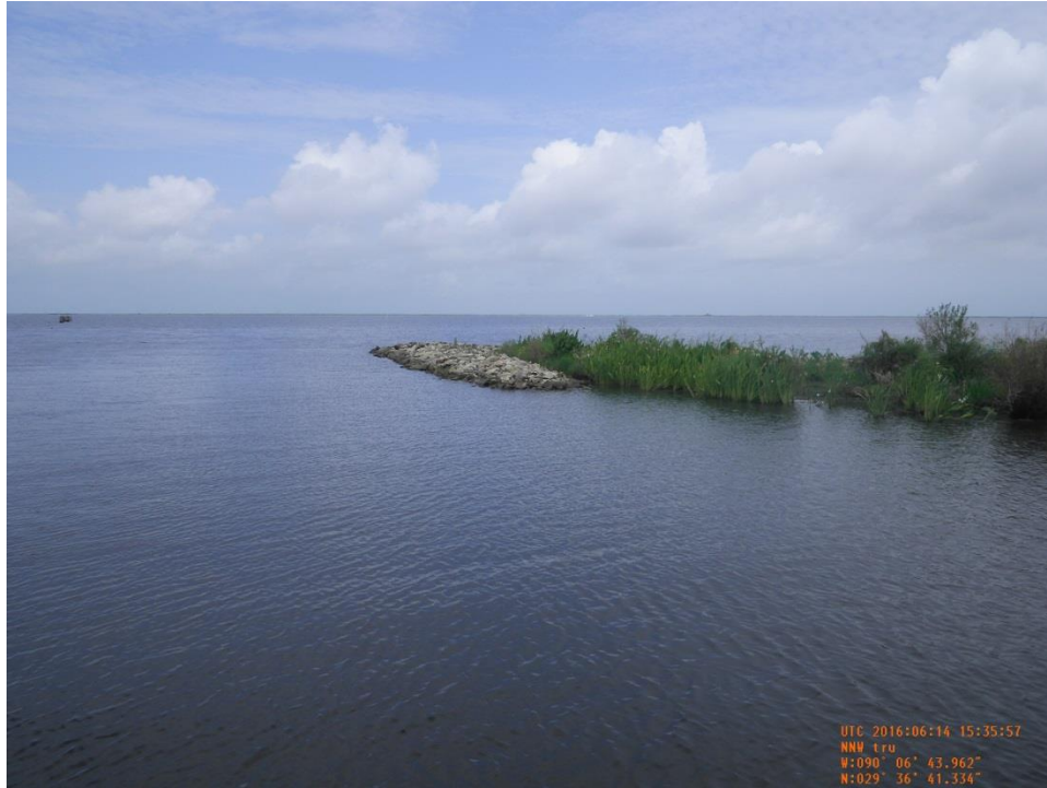
Photo 35: CU#6 rock revetment tie-in to bank at existing canal near Sta. 0+00.
