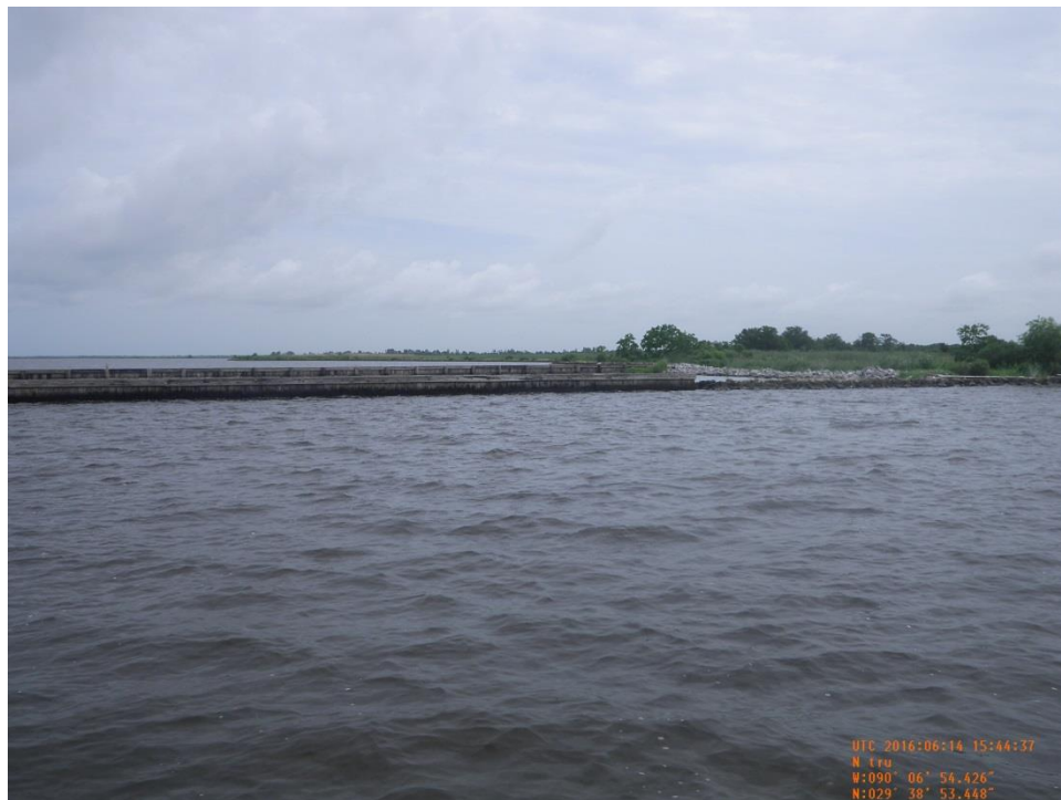
Photo 42: CU#6 rock revetment tie-in to timber bulkhead near Sta. 200+00.
