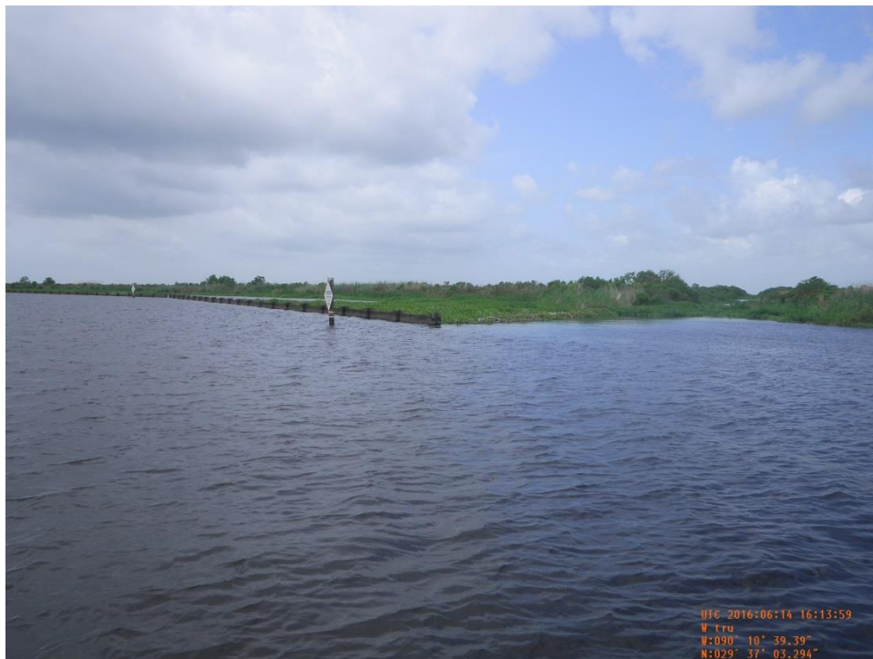
Photo 48: CU#5 rock revetment to rock tie-in near beginning of project.
