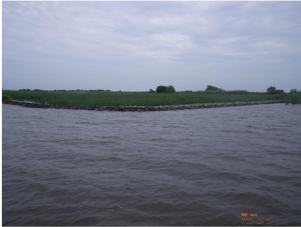
Photo 1: View of the rock revetment (CU#3) along the east bank of Little Lake near Sta. 106+00
