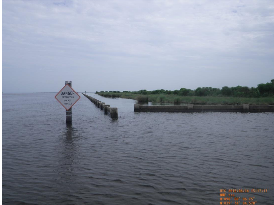
Photo 27: CU#4 Concrete wall (Reach 1) at the Chevron Pipeline along east bank of Harvey Cutoff Canal.
