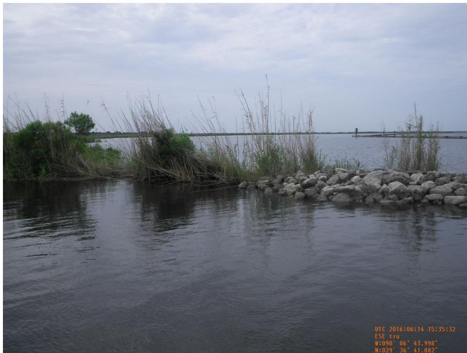
Photo 34: CU#4 rock revetment tie-in to an existing canal bank at the beginning of Reach 1.
