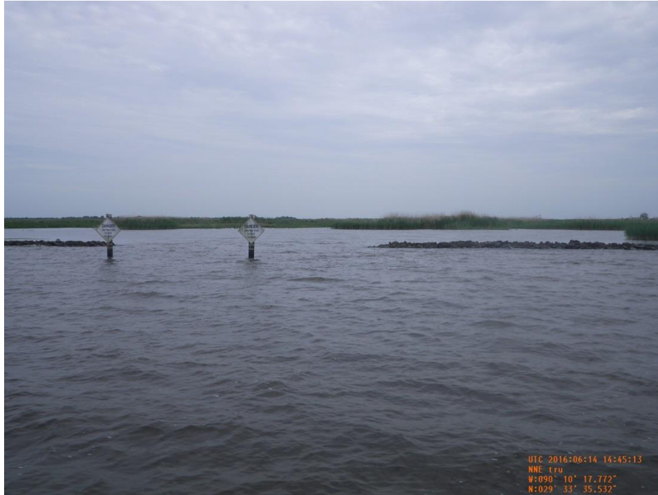
Photo 5: View of fish dip in rock revetment (CU#3) near Sta. 43+00
