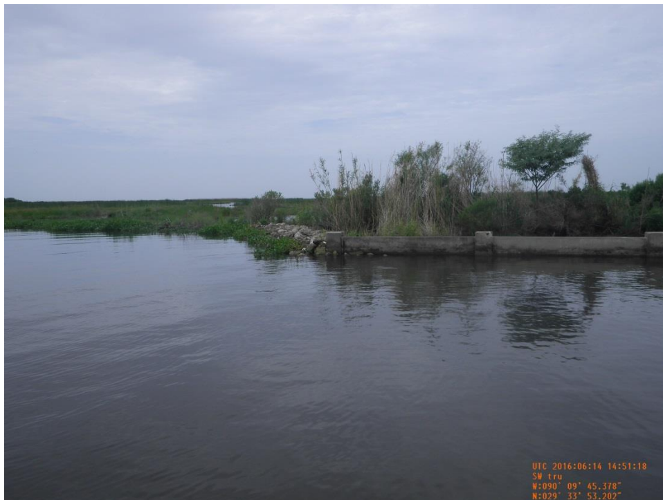
Photo 10: CU#4 Rock revetment closure along south bank of unnamed canal.
