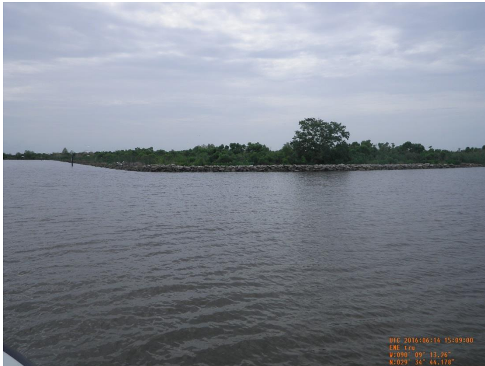
Photo 18: Rock revetment (CU#2 – east side) along south bank of Bayou Rigolettes near mouth of unnamed canal at Sta. 3+00.
