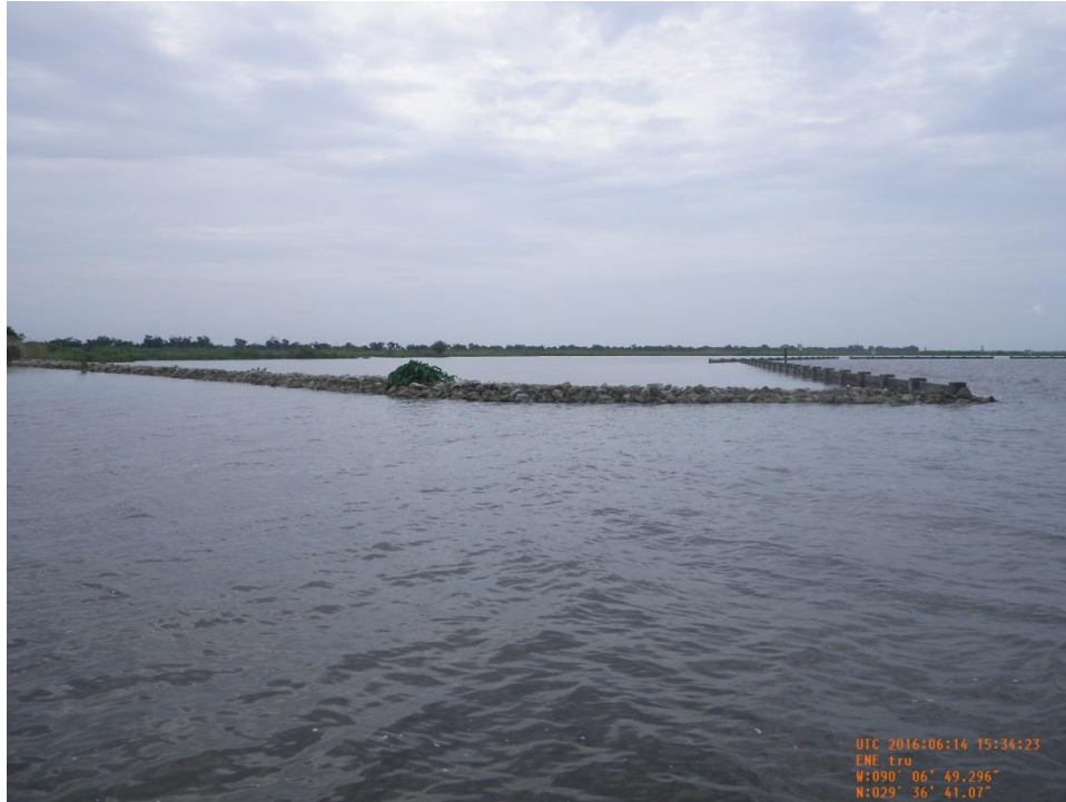
Photo 33: CU#4 Rock revetment to concrete wall (Reach 1) tie-in near an existing canal.
