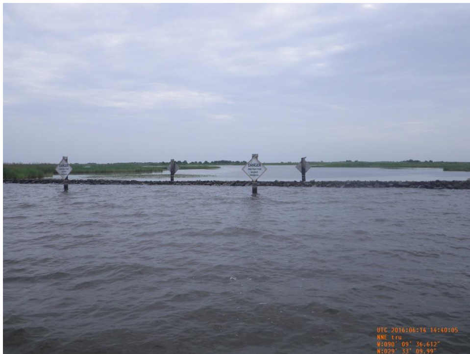
Photo 2: View of rock revetment (CU#3) crossing the opening in the marsh near Sta. 96+00.
