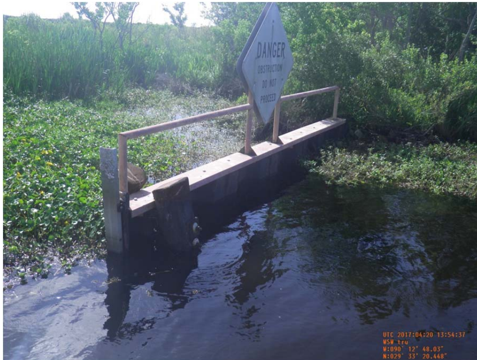
Photo No.29 – view of the stop log bay and sheet pile wall tie-in to bank on the south side of Structure 35.
