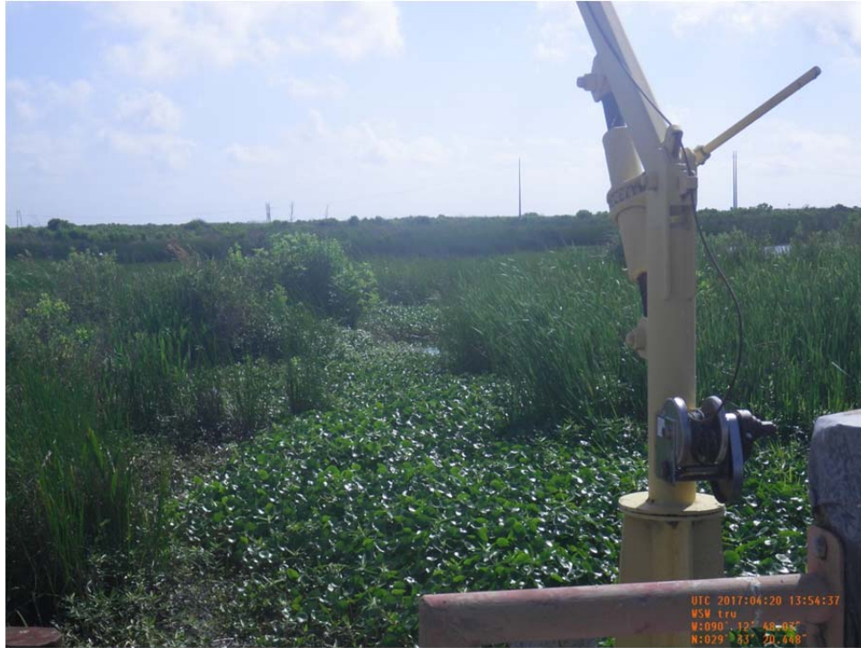
Photo No.27 – view of boom system for moving stop logs and the interior marsh behind Structure 35.
