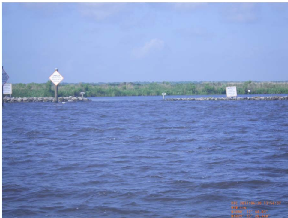
Photo No.16 – view of rock weir with boat bay at Structure 2 from Bay L' Ours.
