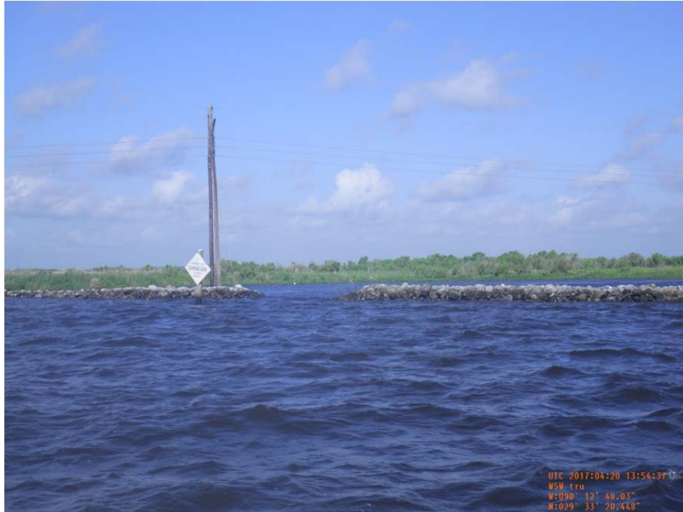
Photo No.13 – view of the warning sign at the fish dip along the rock closure structure between Structures 4A/4B and 4.
