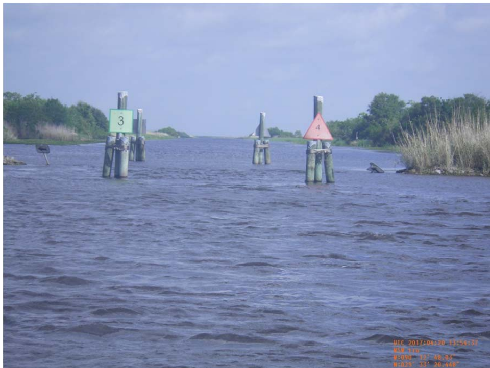
Photo No.36 – view of timber pile dolphins and signs at the entrance to the barge bay at Structure 1.
