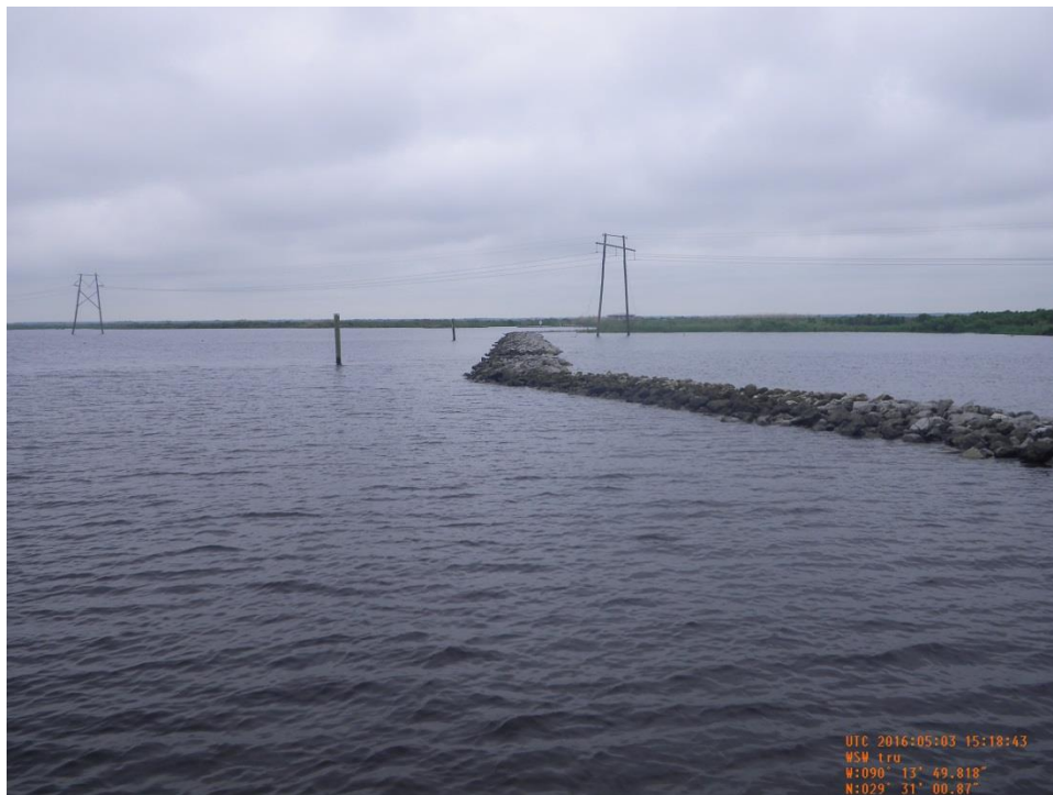
Photo 14: View of rock dike closure between Structure No.4B and Structure No.4 constructed in 2012.
