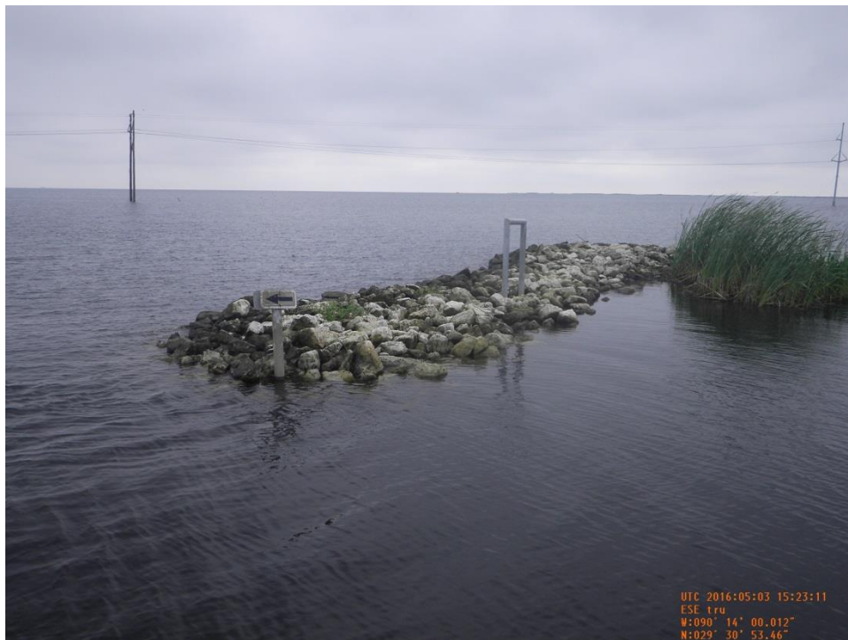
Photo 20: View of the rock weir on the south side of the boat bay of Structure No.4.
