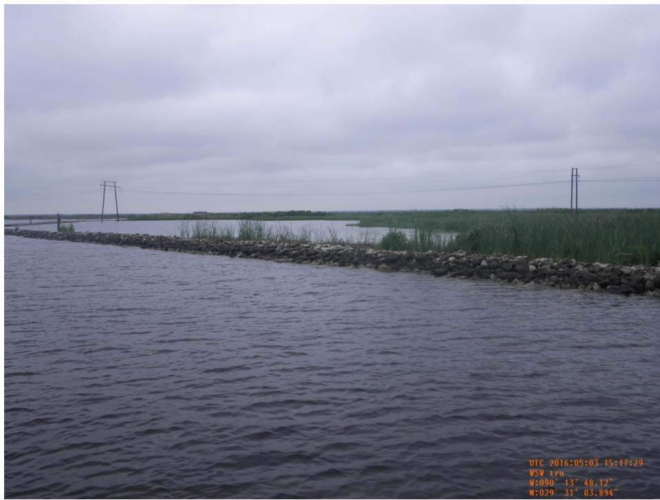
Photo 12: rock plug (Structure 4A & 4B) and rock dike extension to Structure 4 construction in 2012.
