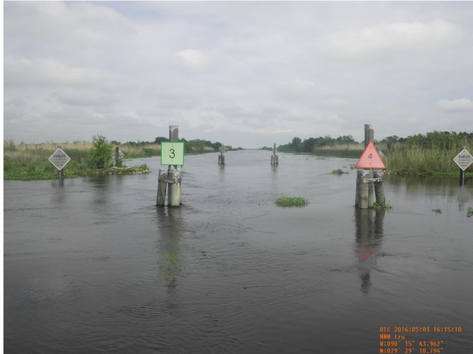
Photo 37: View of rock weir on the west side, warning signs and barge bay opening at Structure No.1 located along Superior Canal.
