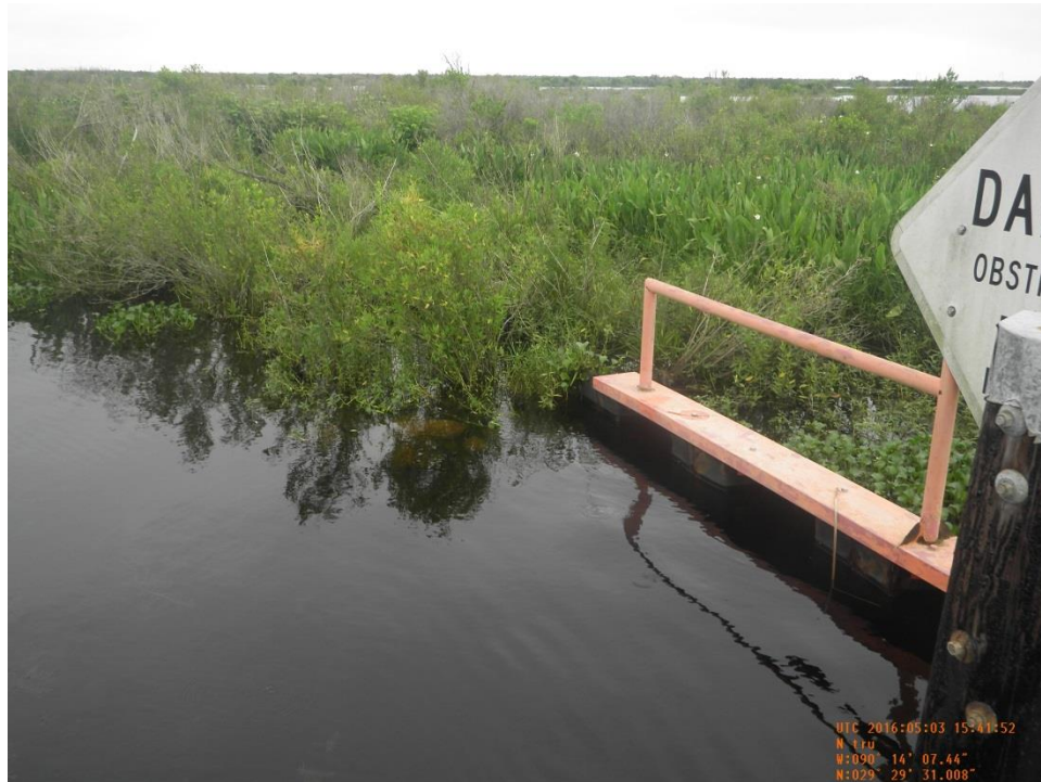
Photo 27: View of steel sheet pile weir and bank tie-in on the NE side of Structure No.35.
