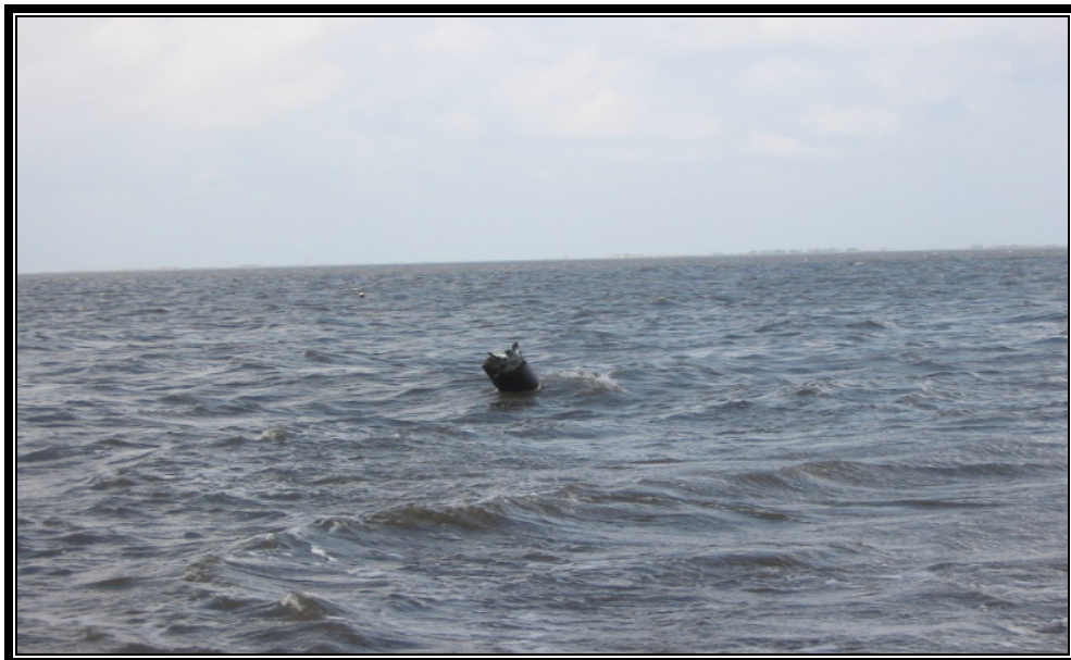
Timber pile cluster after damage showing batter pile protruding from waters surface.
