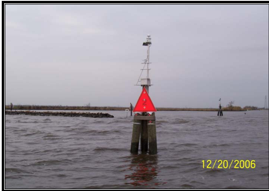
Replacement of timer pile cluster and navigational aid lights and signage.
