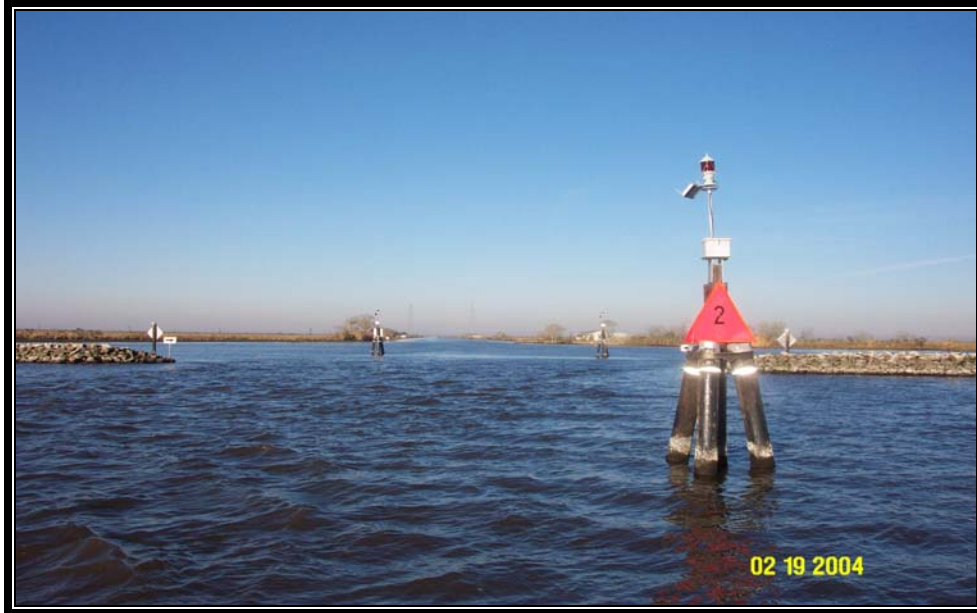
Photo of timber pile cluster and navigation light prior to being destroyed.
