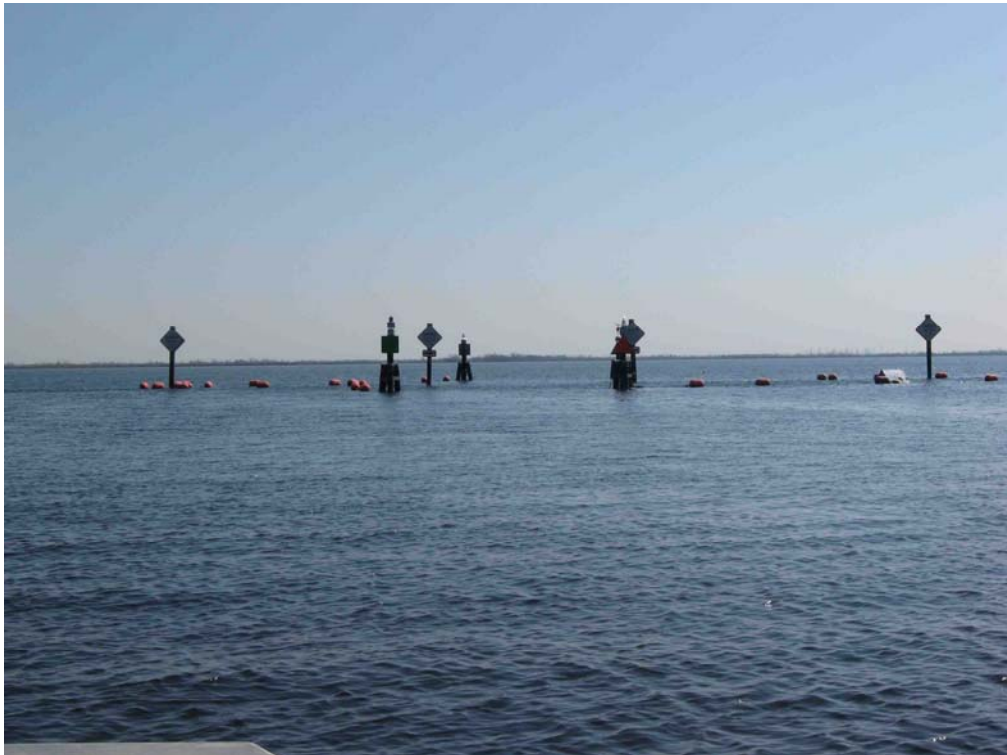
Photo #2 – Goose Bayou Canal Weir. Looking East toward the Pen.
