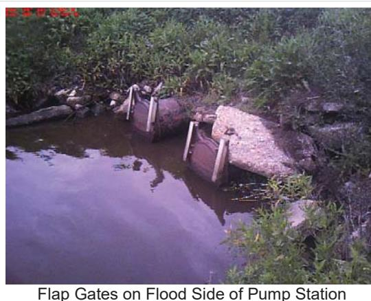
Flap Gates on Flood Side of Pump Station
