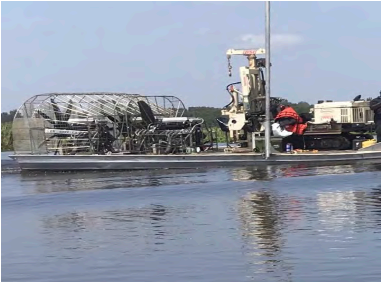
Figure.2: Airboat Mounted Drill rig
