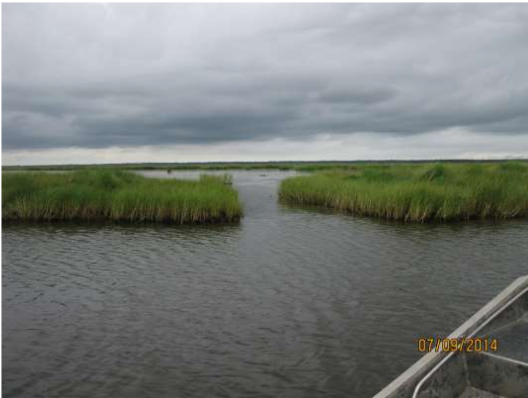
Area A – Containment degraded for tidal exchange at north end of fill area
