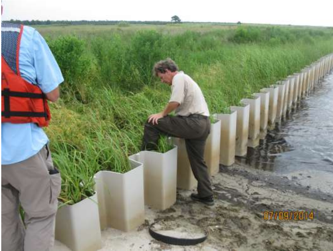
Area D – Marsh infill behind vinyl sheet pile wall
