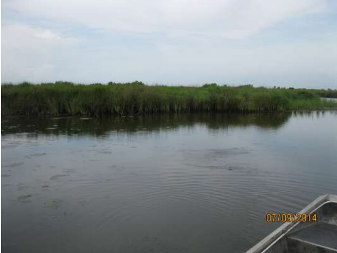
Area B – Shallow water in containment borrow area with fill area beyond
