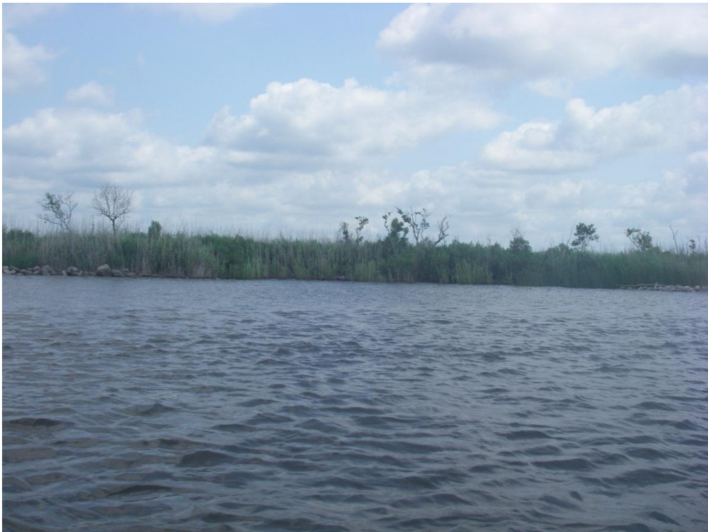
Photo No. 2, Low Area of Displaced Rock Dike
