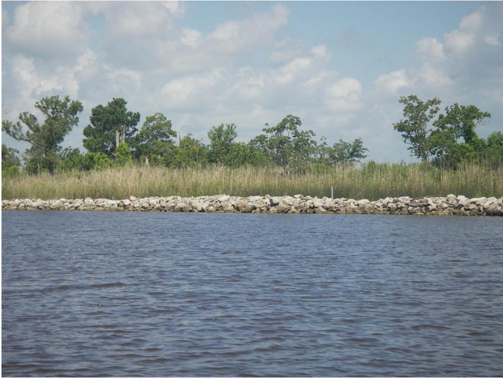
Photo No. 1, Typical Rock Dike
