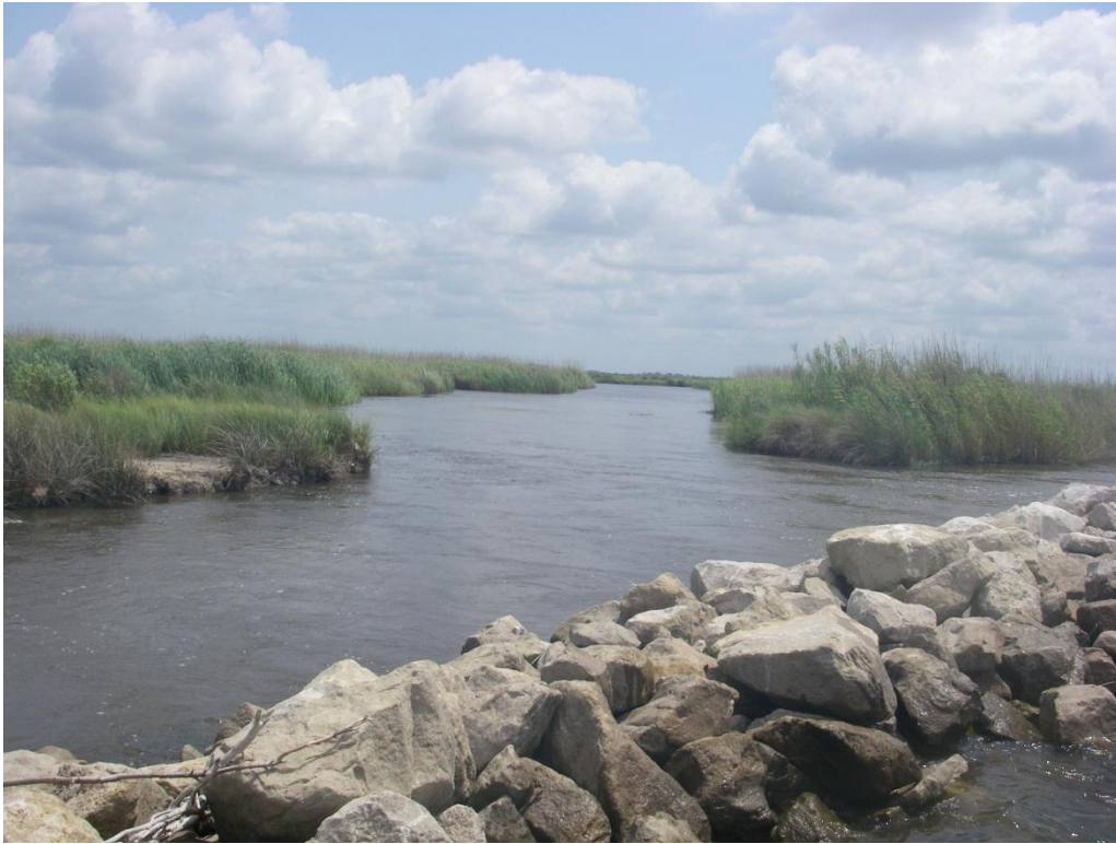
Photo No. 3, Gap in Earthen Plug behind Rock Dike, Water Flow Channeling into Marsh
