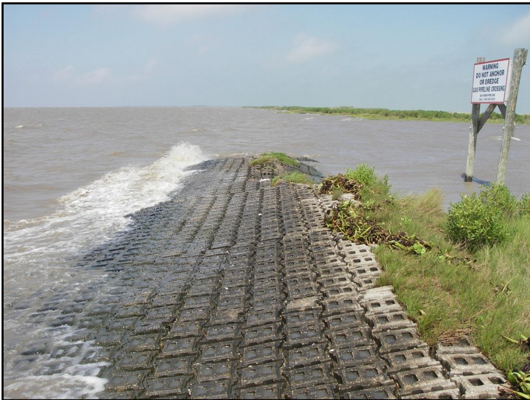
Photo 2, Area 2, West side of concrete mats.
