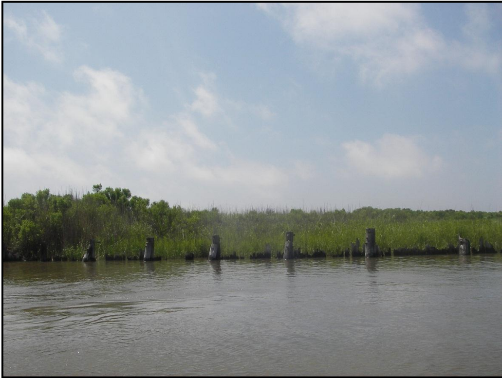
Photo 1, Area 1, Timber bulkhead.
