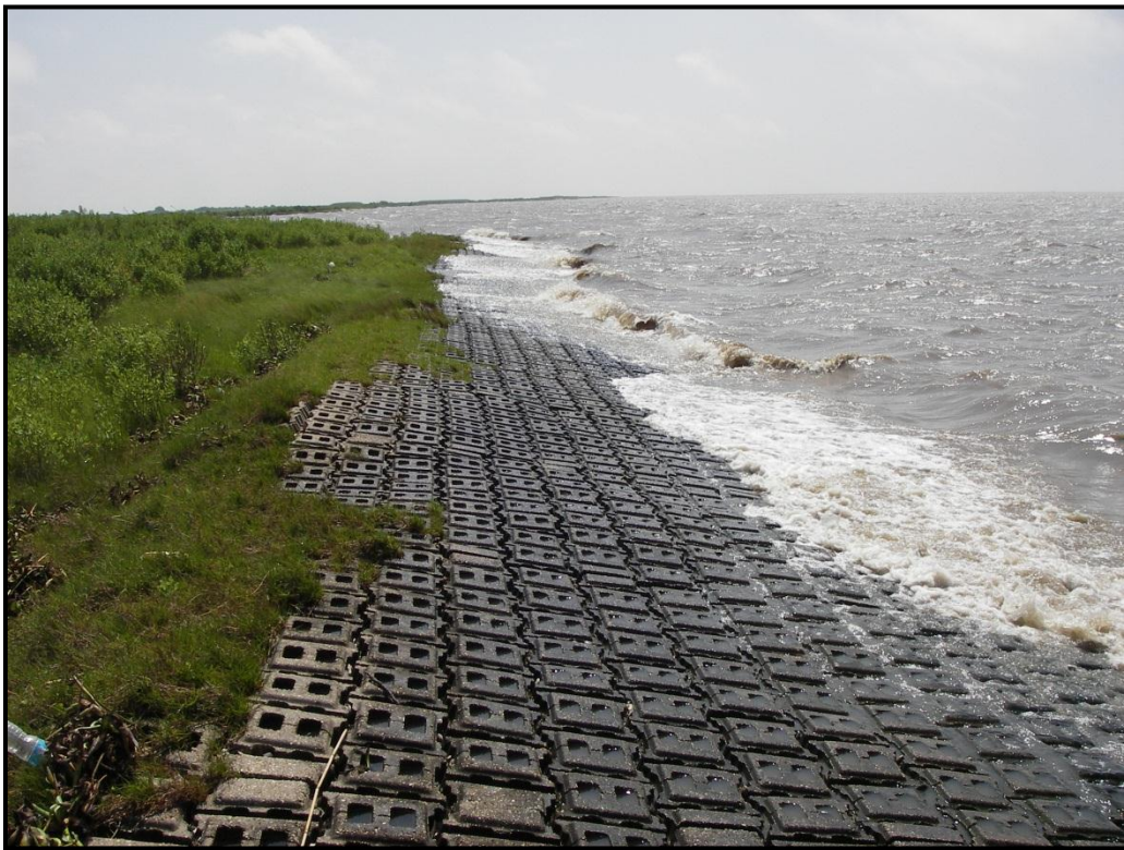
Photo 4, Area 2, East side of concrete mats.
