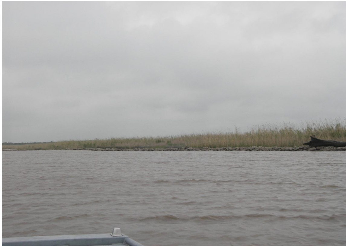
Photo No. 2 —typical reach of dike
