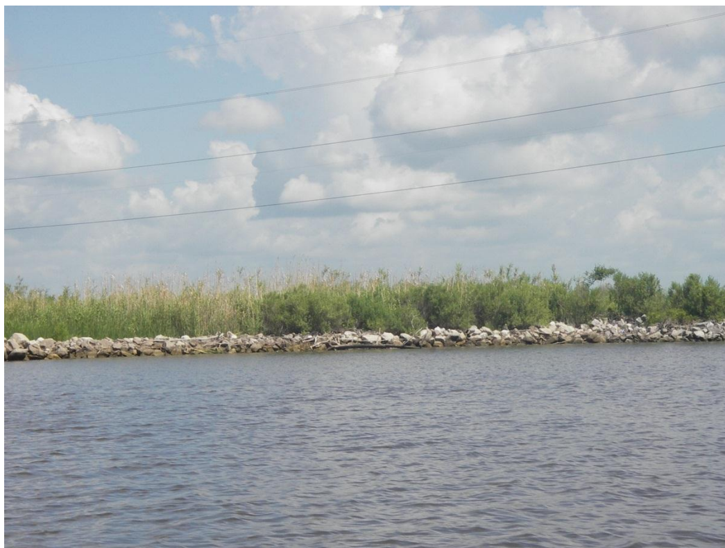
Photo No.1 , Typical Rock Dike
