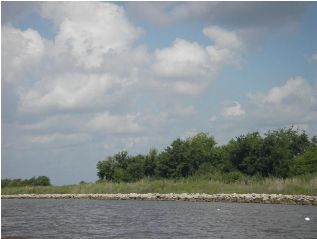
Photo No. 2, Vegetation behind Rock Dike
