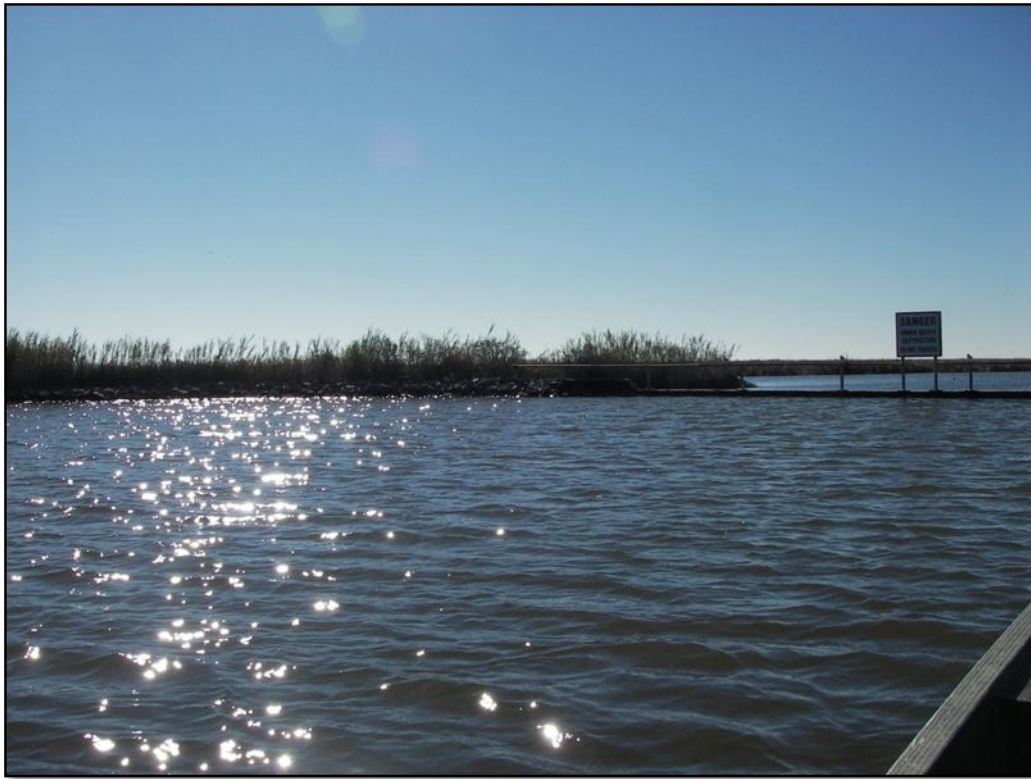
Photo 7, Mangrove Weir, view of rock armor east side.
