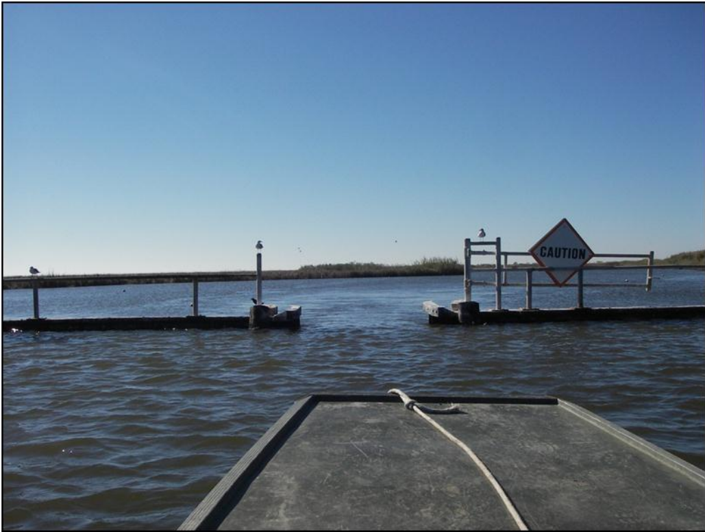
Photo 5 , Mangrove Weir, view looking south.
