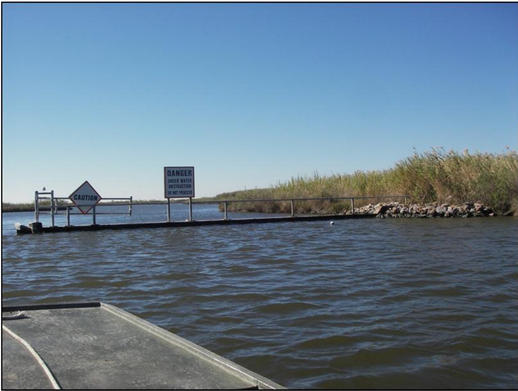
Photo 6 , Mangrove Weir, view of rock armor west side.
