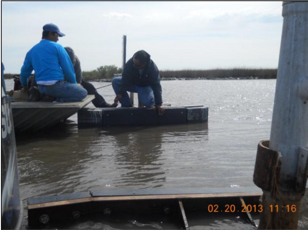
Photo 4 , Grand Bayou Weir, boat guide replacement.
