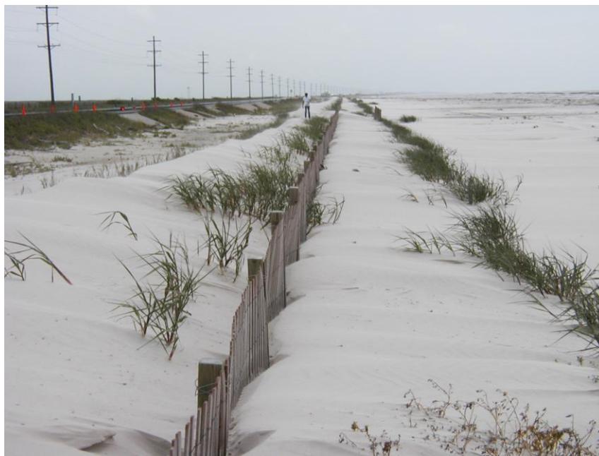
Figure 9a. View of the sand fencing and Vegetation Plantings at Station CS31-108 taken in April 2004. Note the dune formation almost covering the fences. The photograph is facing east.
