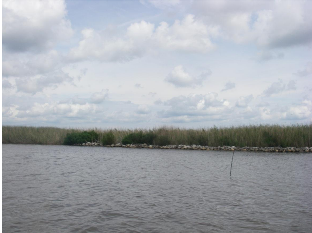
Photo No. 2, Western End of Sweet Lake Rock Dike
