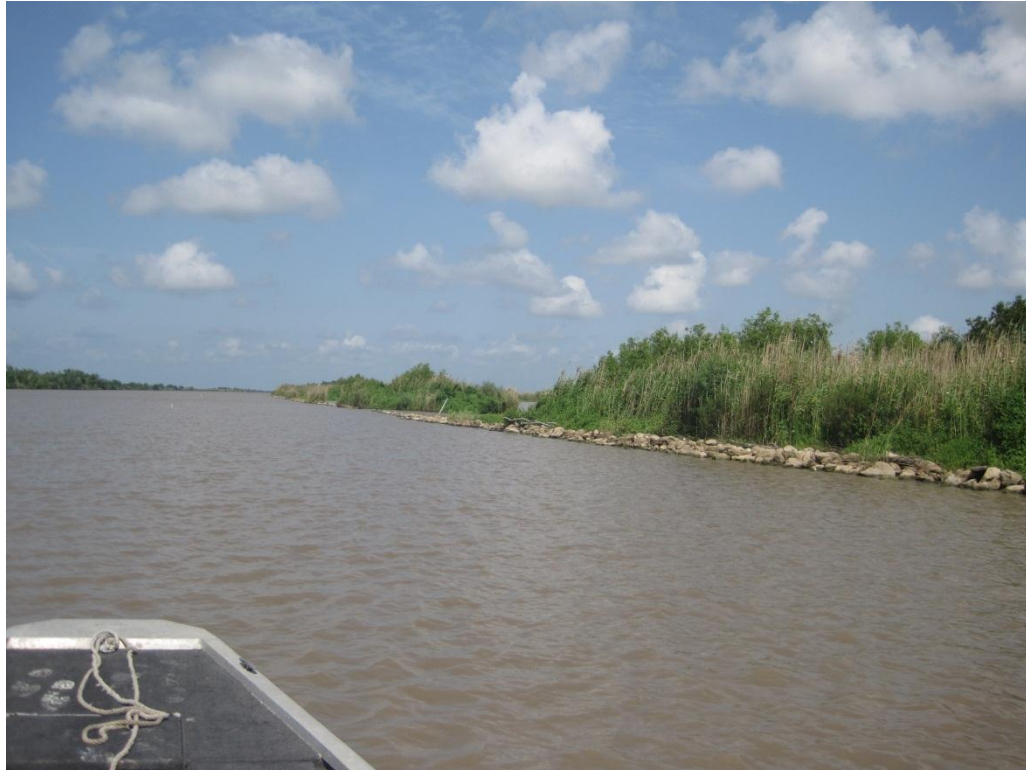
Photo No. 1, (Sweet Lake) Typical rock dike
