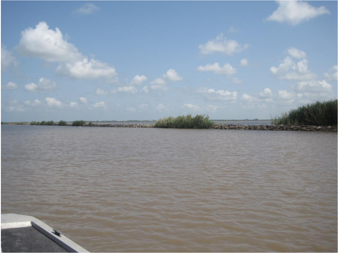
Photo No. 3, Willow Lake Rock Dike (Southeastern End)
