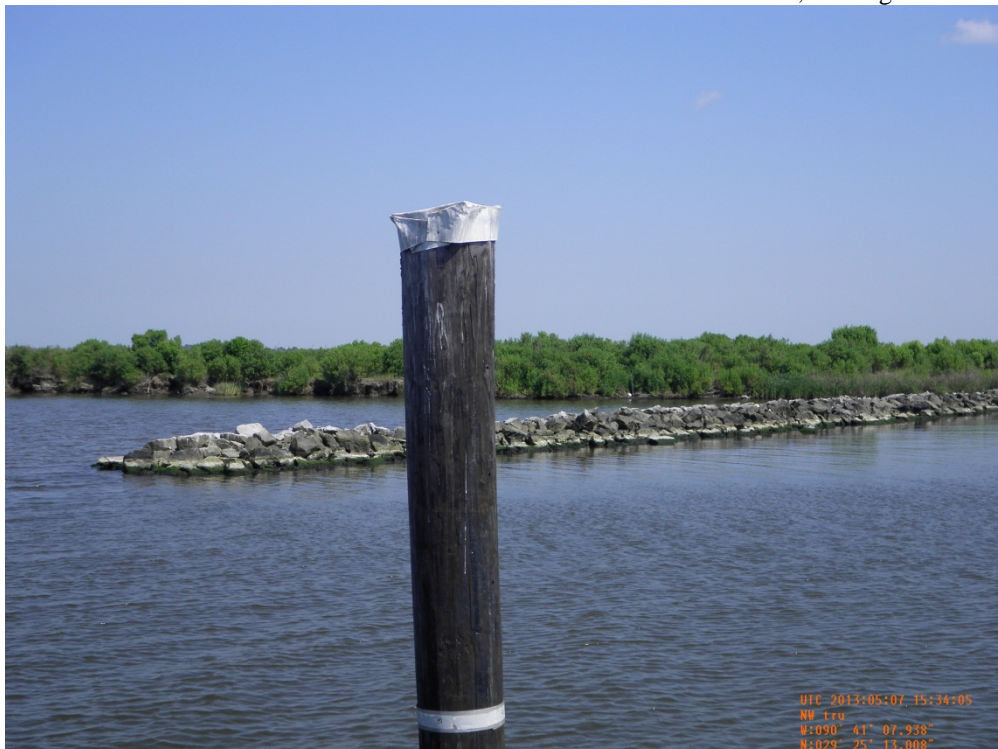
Photo 12: The warning sign on the lake side of the choke down section is missing from its support.
