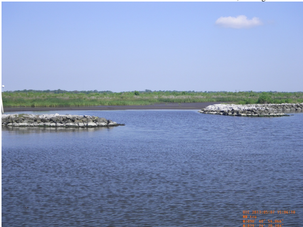
Photo 2: View of access corridor for Gulf South pipeline in foreshore rock dike, looking west
