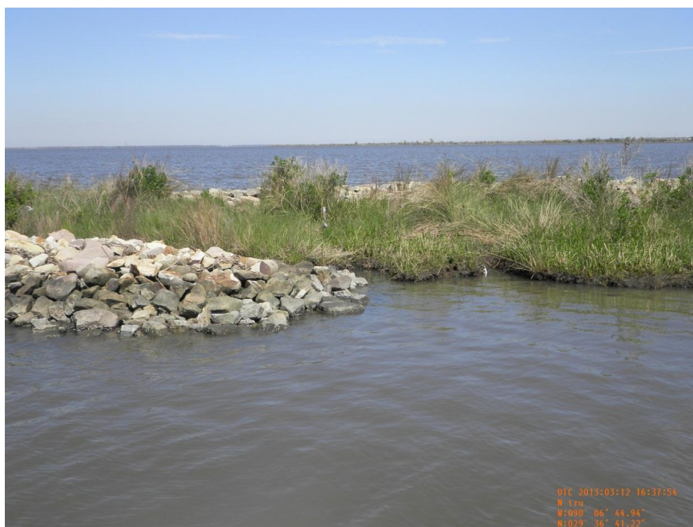
Photo 38: View of CU#6 rock embankment tie-in on north side of oilfield canal
